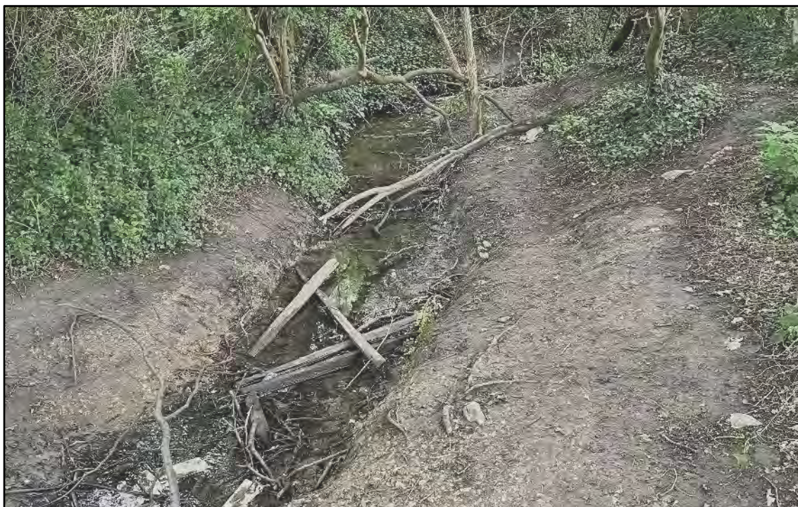
Figure 2-3: West Brook watercourse, north of Coldharbour Farm Road and adjacent to the proposed development site (02/07/2021)
