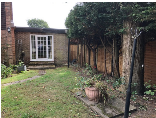
Rear View on Extension
