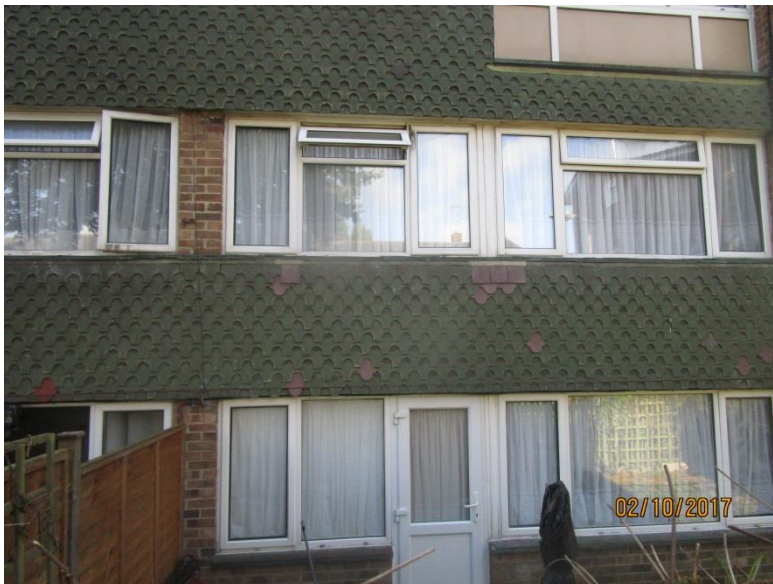
Photo 5 - Tile hanging to front elevation
