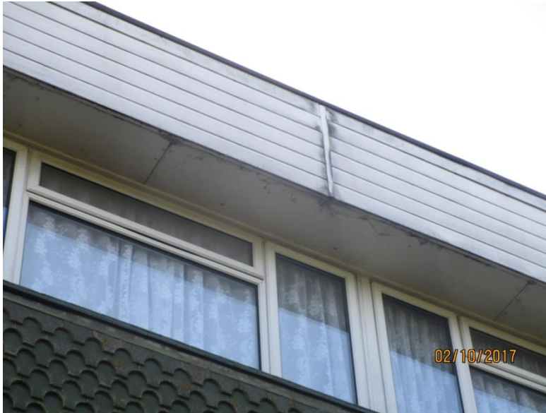
Photo 4 - Existing Fascia Board and Soffit
