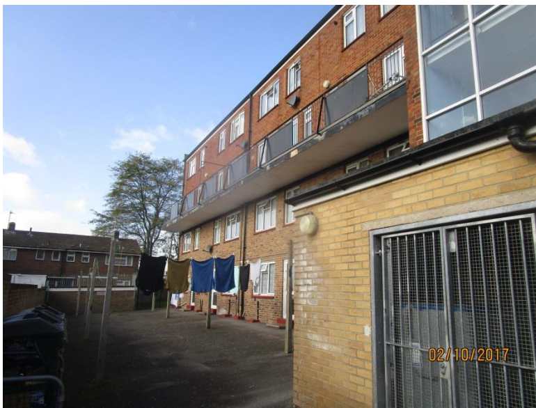
Photo 3 - Rear elevation showing balcony walkway
