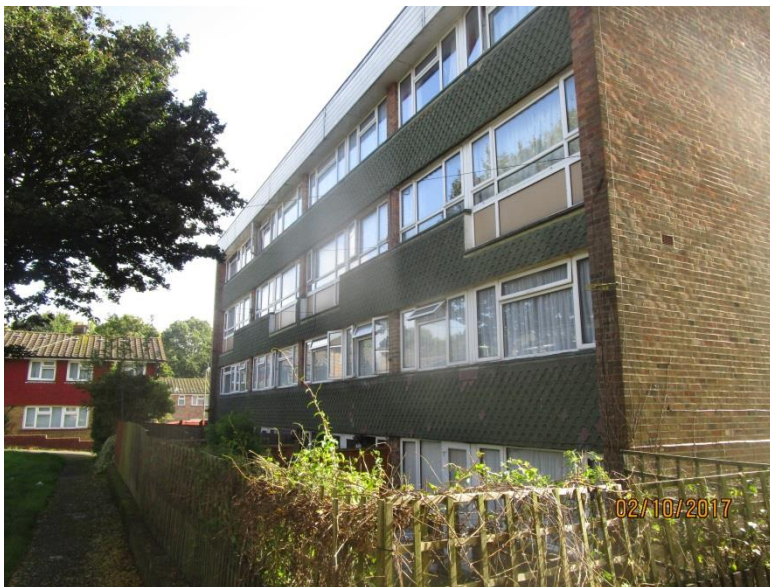
Photo 2 - Front Elevation showing boundary fencing
