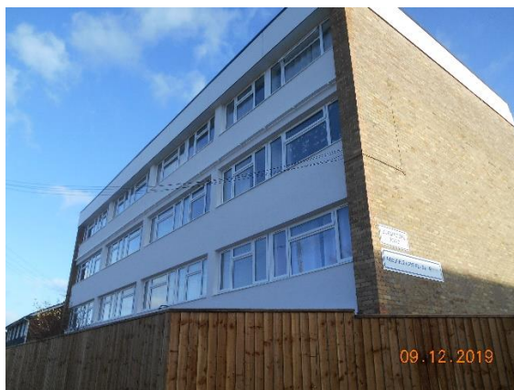
Similar Completed Pilot Block (Prospect Lane)
