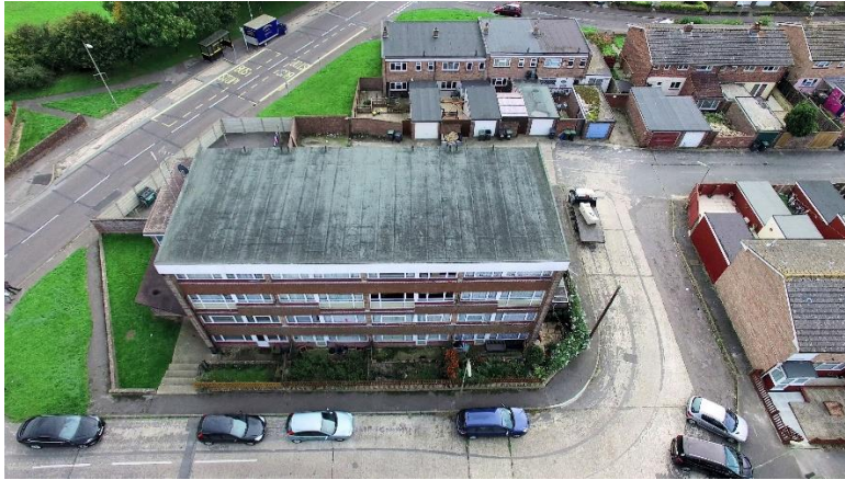
Photo 1 - Arial view of the block (Front Elevation)
