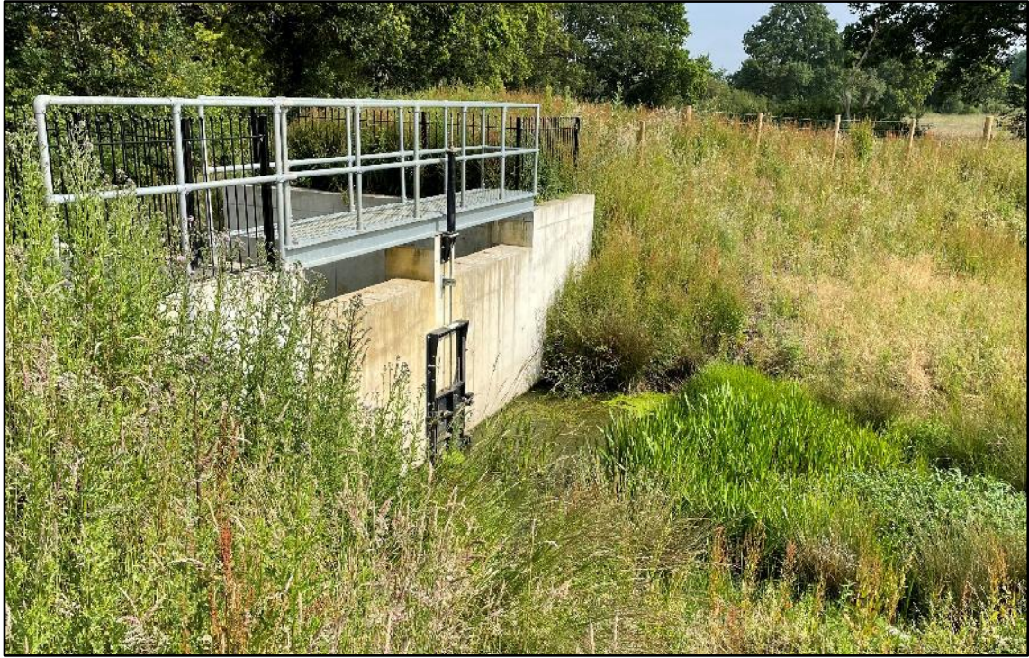
Figure 2-6: Flood attenuation area control structure (02/07/2021)
