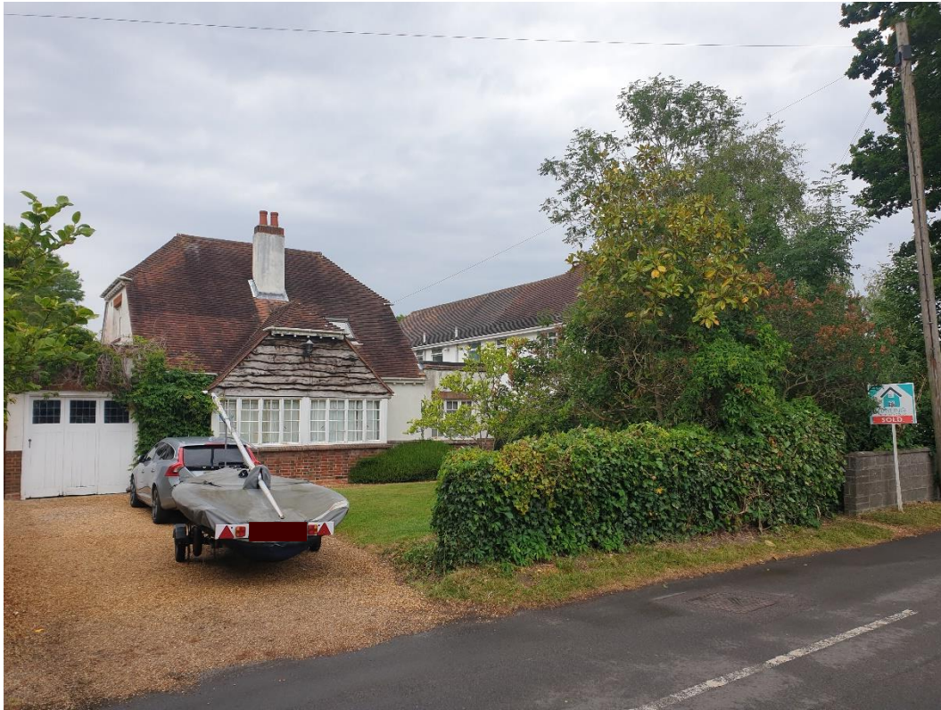
48 Sinah Lane – Front view
