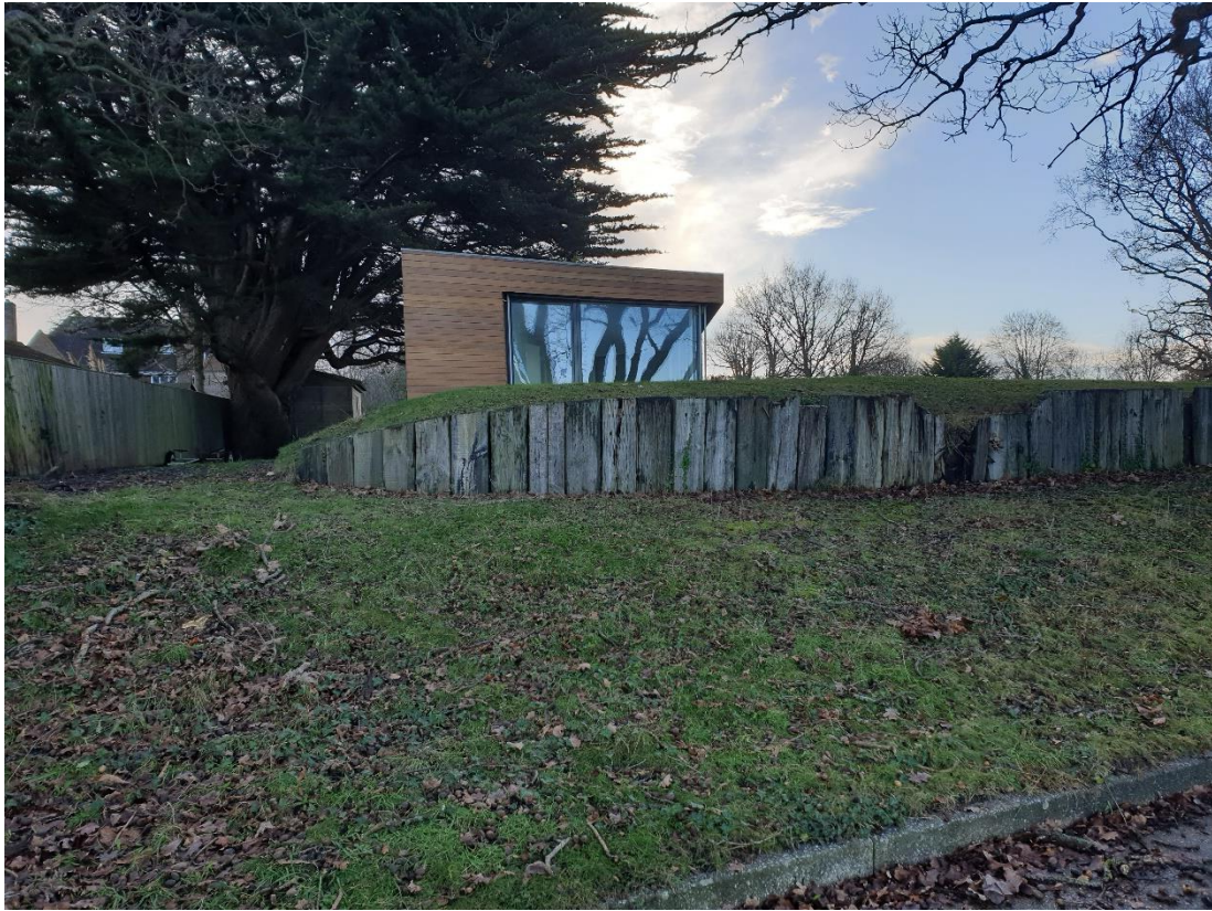
a. No. 40 Sinah Lane Outbuilding
