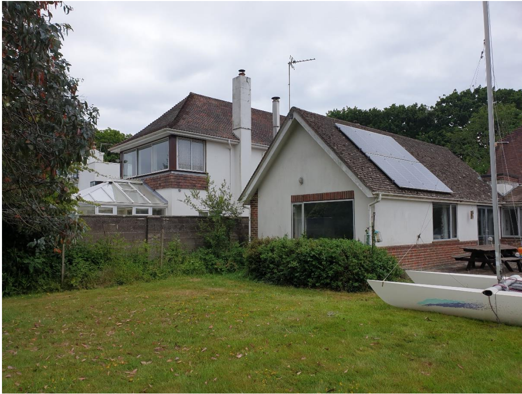
View towards 46 Sinah Lane (rear)
