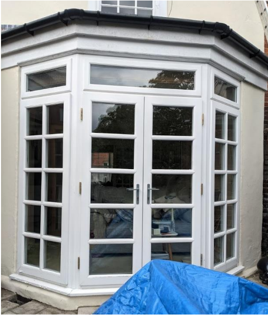
(Photograph 7 – Existing dining room bay windows)
