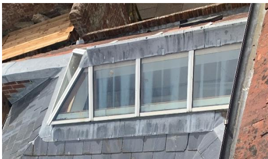
(Photograph 10 – Existing kitchen roof lantern)
