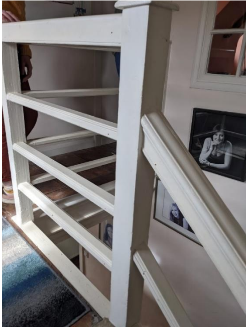
(Photograph 14 – Existing stair balustrade at second floor – to be replaced)
