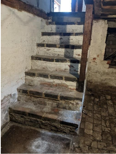
(Photograph 1 – Existing basement stair)
