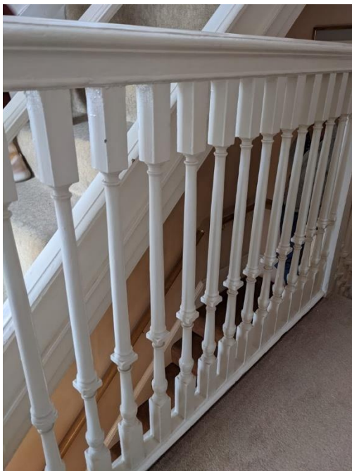
(Photograph 15 – Existing stair balustrade at first floor – to be replicated at second floor)
