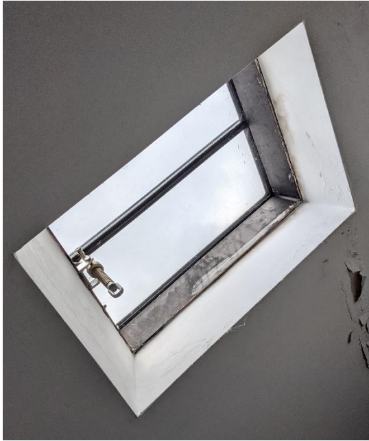
(Photograph 4 – Existing utility roof light)
