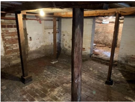
(Photograph 2 – Existing main basement area)
