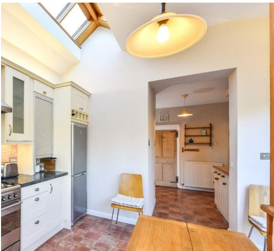
(Photograph 8 – Existing opening between the hallway and kitchen – to be enlarged)
