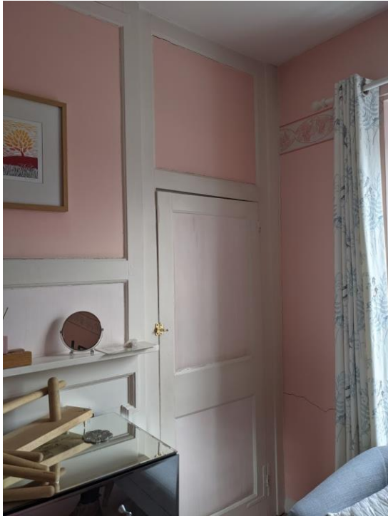
(Photograph 12 – Existing cupboard in bedroom 2)
