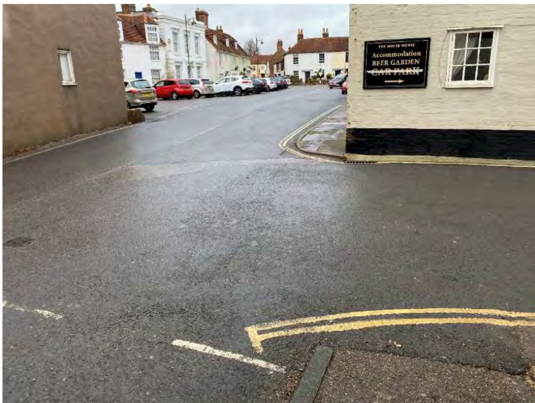
Image 32: Lack of Tactile Paving over New Road
