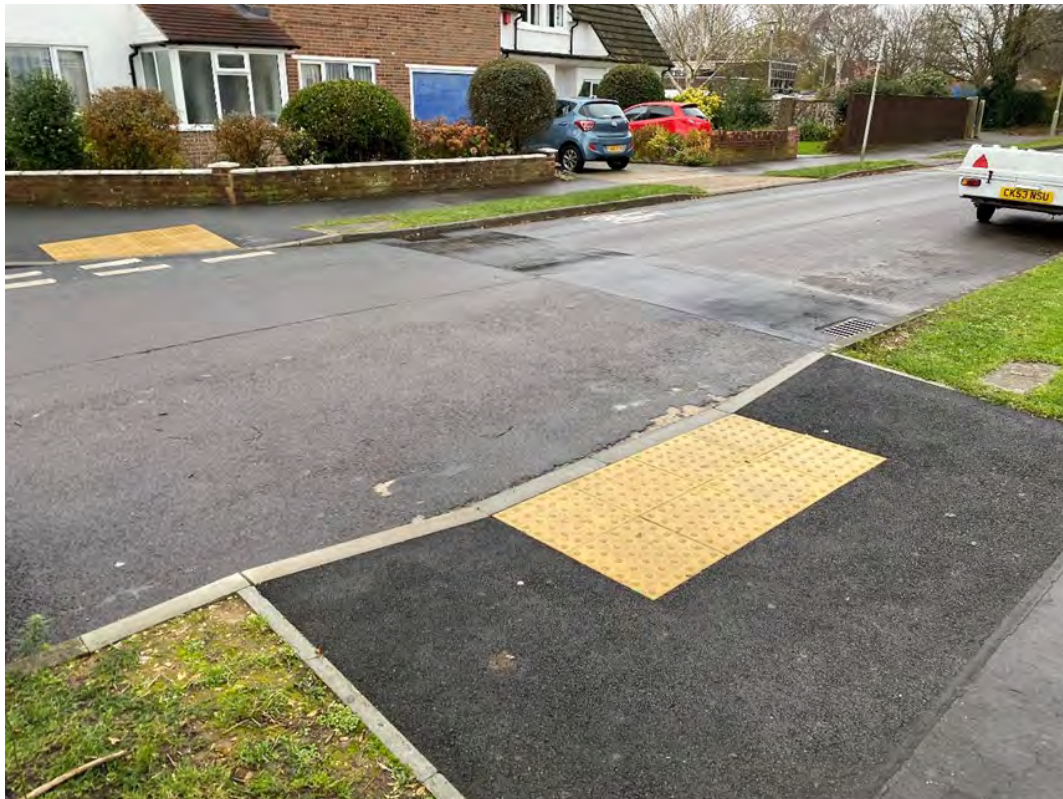
Image 6: Dropped Kerb and Tactile Paving to reach Primary School
