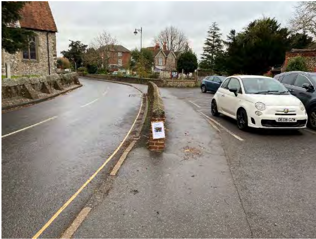
Image 32: Lack of Tactile Paving over New Road
