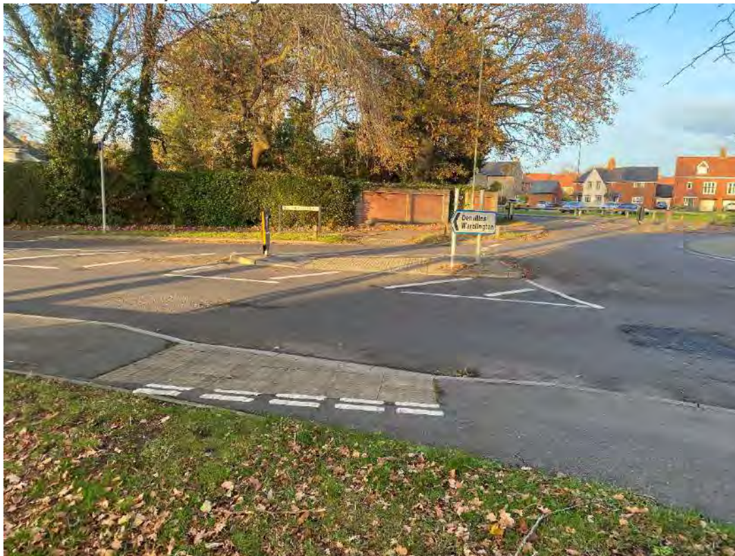
Image 14: Pedestrian Crossing Point (western arm) – Redlands Lane / New Brighton Road / Westbourne Road / Southleigh Road Roundabout
