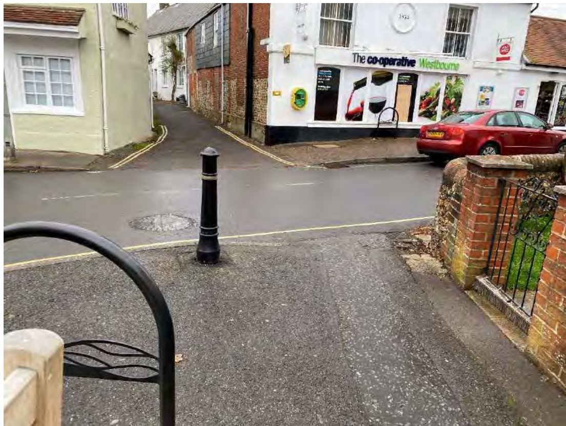
Image 33: Lack of Tactile Paving over The Square
