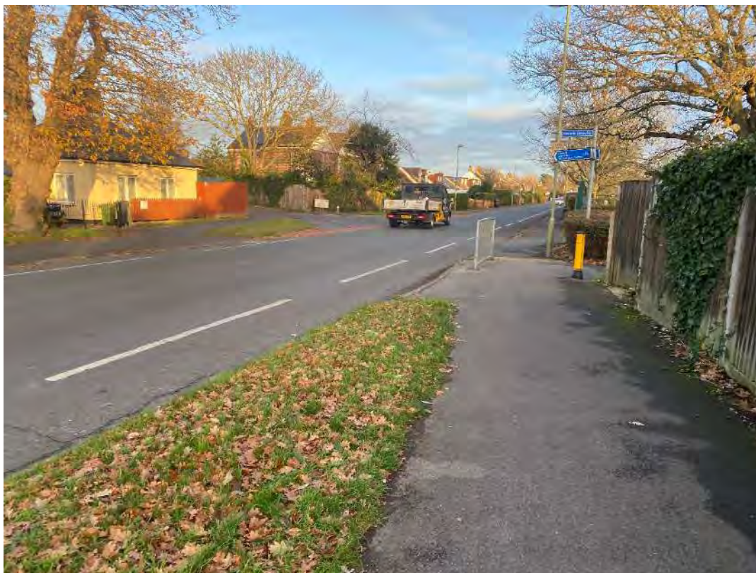
Image 8: No tactile paving at crossing on Southleigh Road near Hollybank Lane
