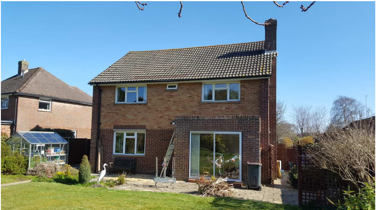
Photo of the rear of the existing house.
