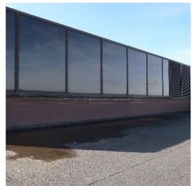
Detrimental pooling and patchwork of flat roofing repairs to building 6000
