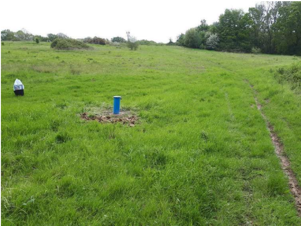
Plate 3: Borehole installation at WS1 with raised cover.
