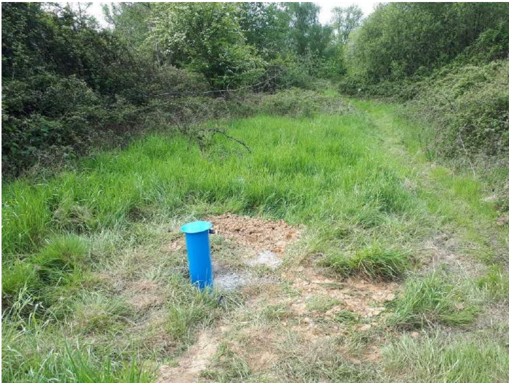
Plate 9: Borehole installation at WS5 with raised cover.
