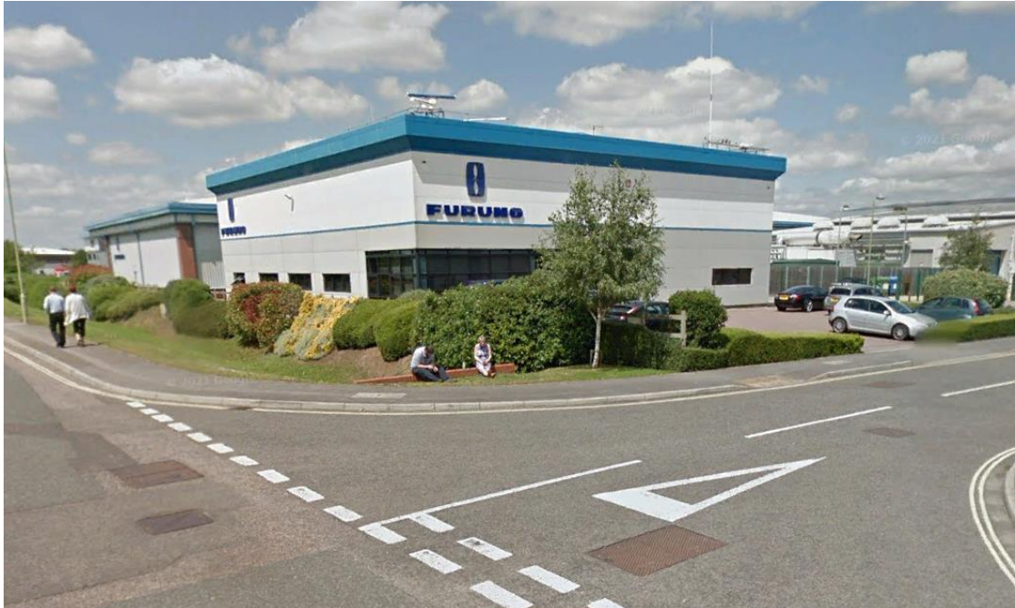
Photo.1 – Building viewed from the south-east (source Google Streetview)
