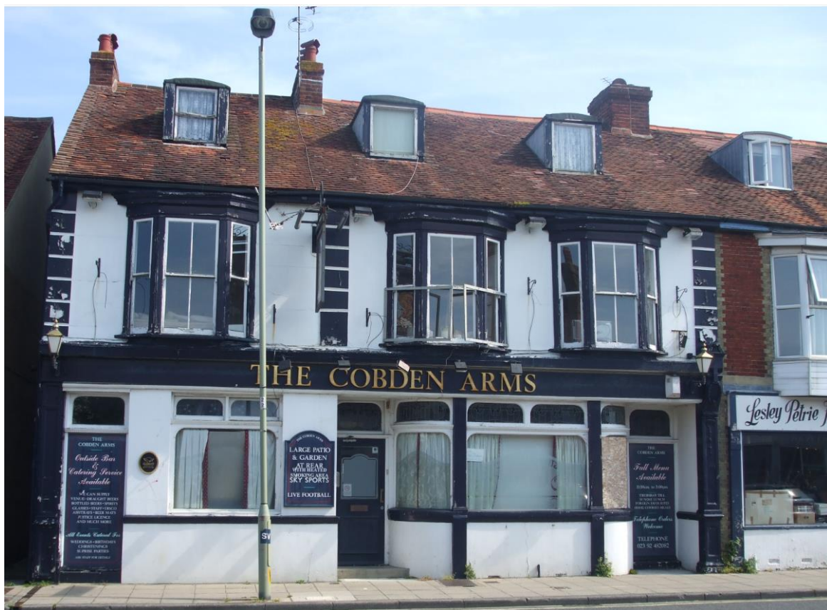
Above: South Elevation of the Cobden Arms Prior to Conversion
