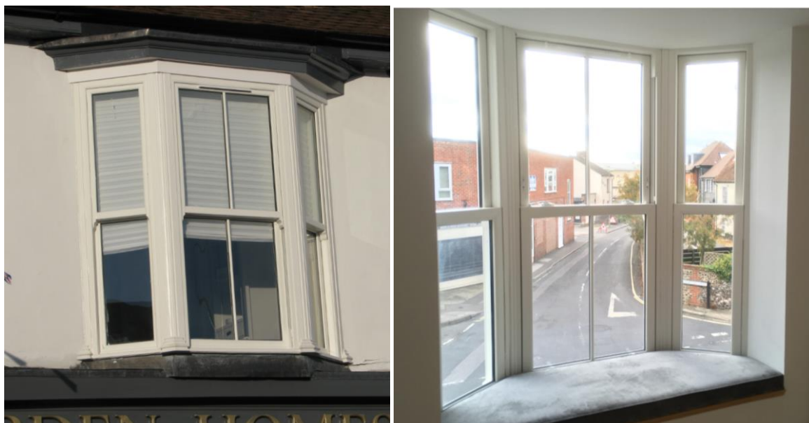
Above: Close Up Photograph of Replacement UPVC Sliding Sash Windows (Exterior and Interior)
