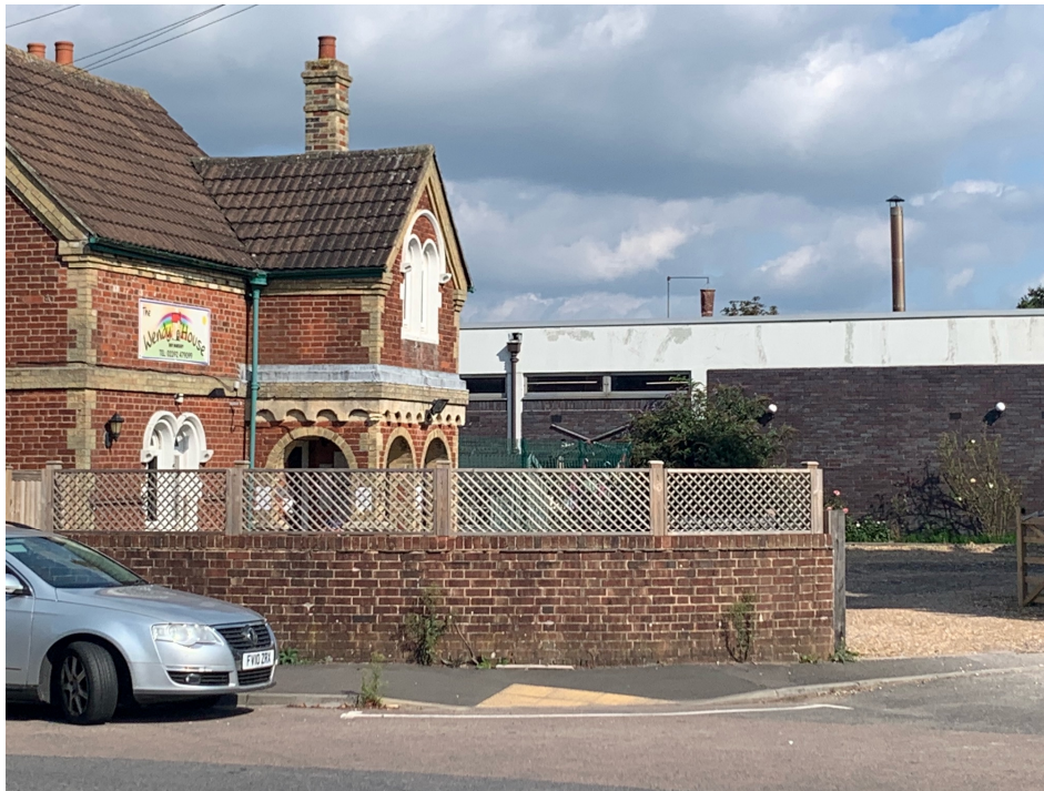
Figure 9: West elevation of Building B with ‘The Wendy House’ in the foreground.
