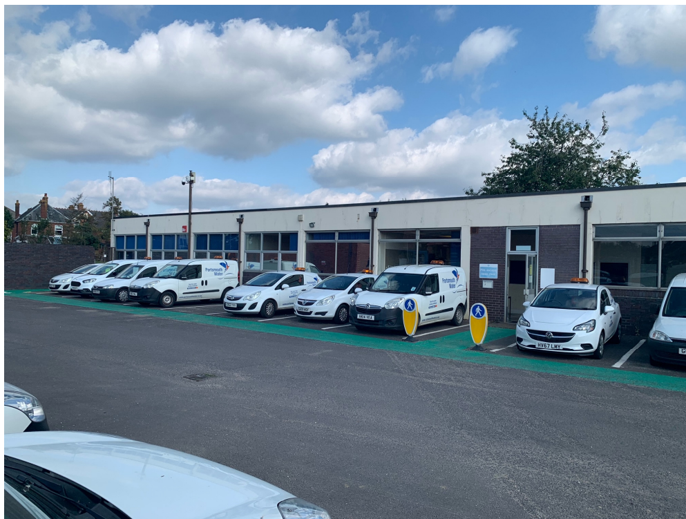
Figure 8: West elevation of Building A.
