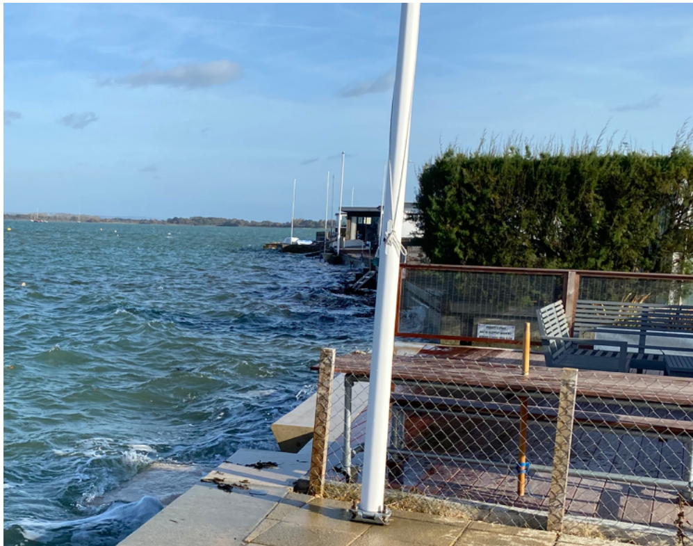
Photo 3 Sea wall and pier/steps looking east on a high tide.
