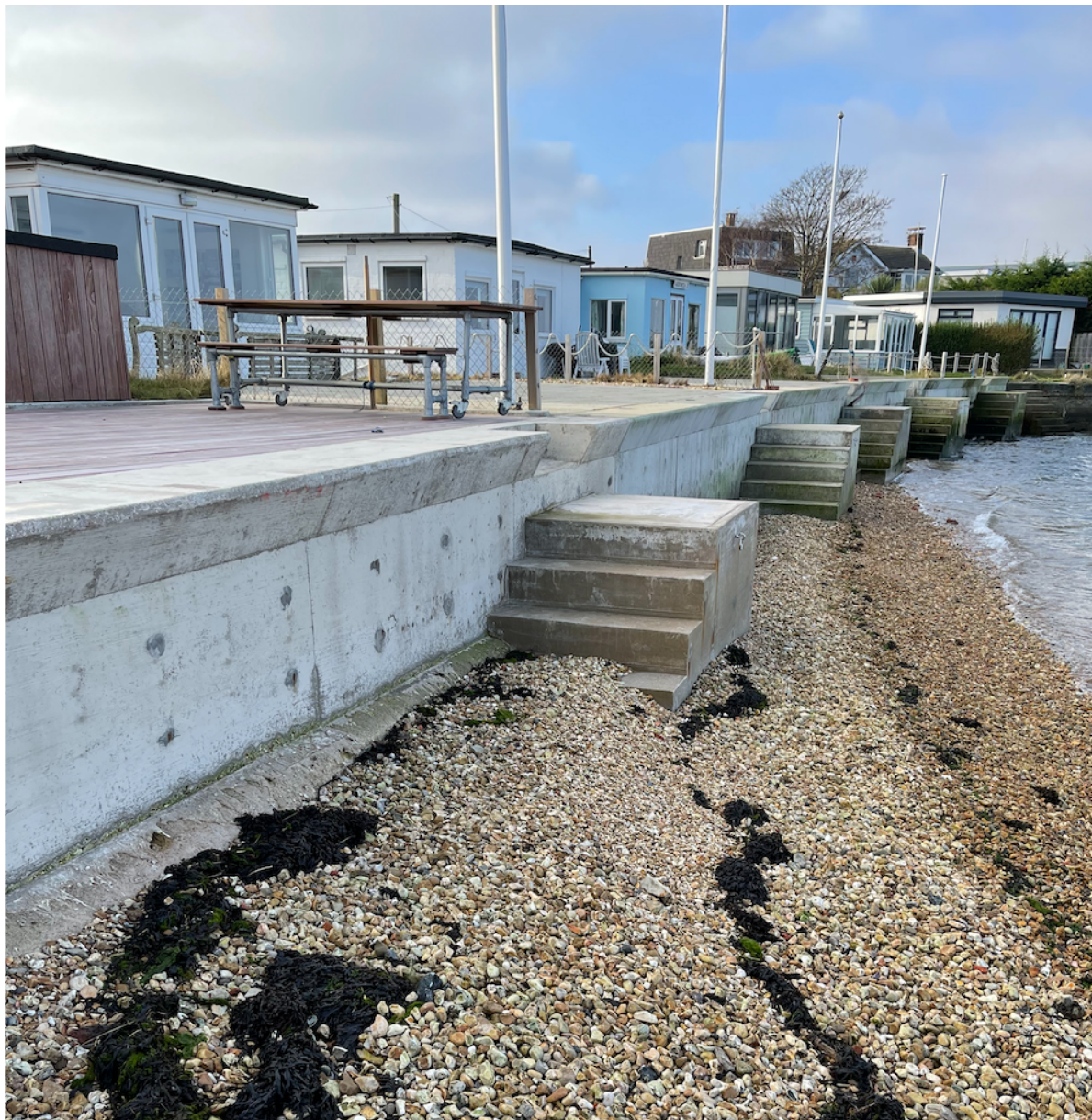
Photo 1: Showing pier / steps to the beach looking west.
