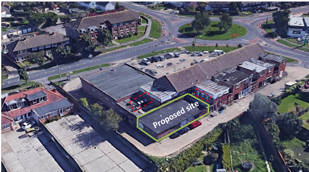
Fig.17 – Photo showing the location of the nearby air-conditioning units.
