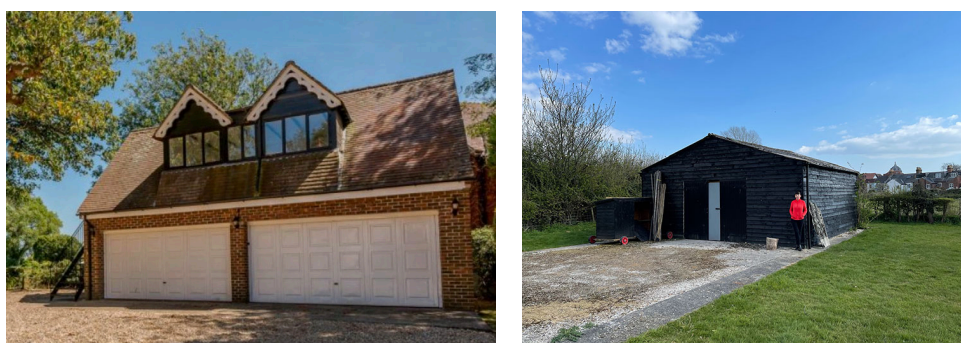
Two double bay garage with studio flat (left) and Shiplap Clad Barn (right)
