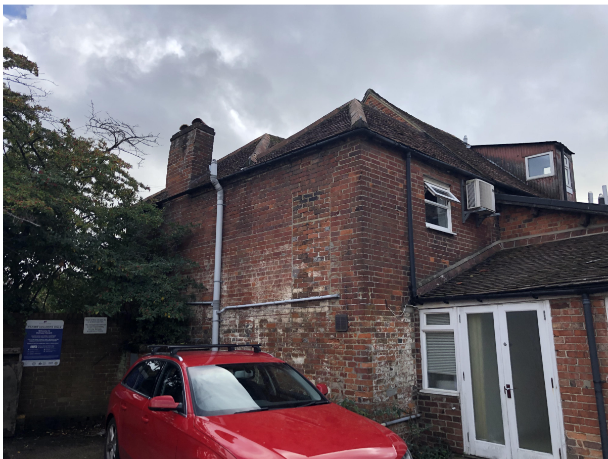
Back view from Waitrose, Havant- yard
