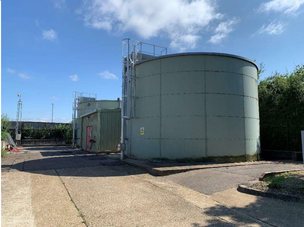
Photograph 5: Water tanks to be demolished
