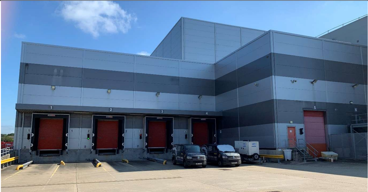
Photograph 3: Elevation of Building D and E (Goods in/ out)
