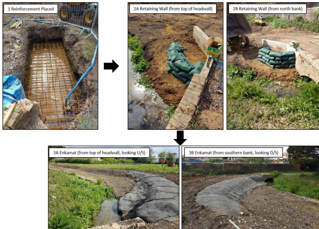
Figure 2: Retaining Wall and Enkamat Construction Process
