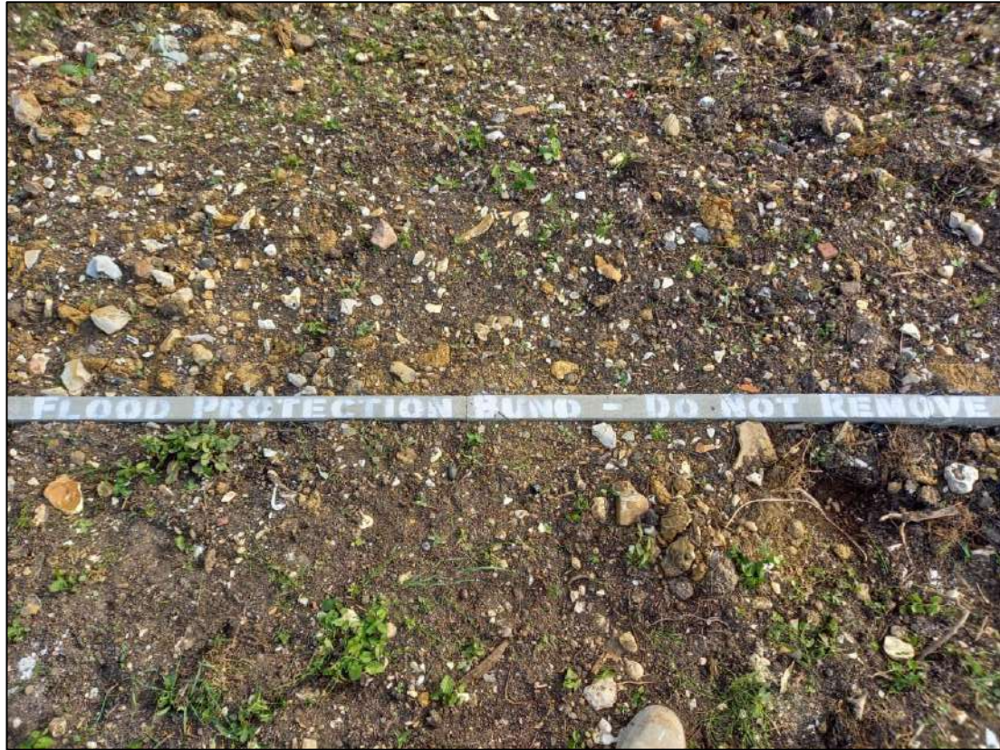
Figure 3: Evidence of Flood Defence Marker on Bund Edging
