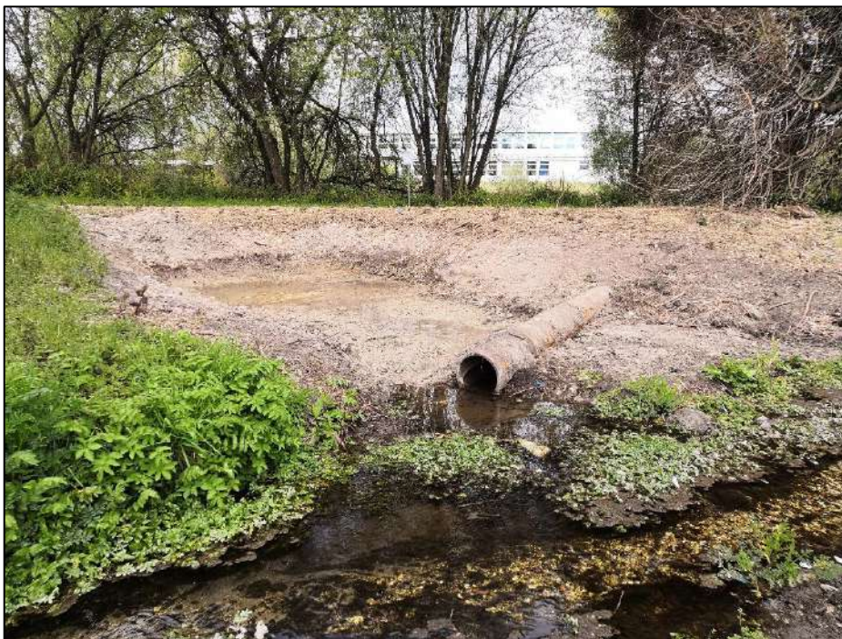
Figure 1: Existing Overflow Pipe in Compensation Area (Ref. Photograph 3 in Report Ref. 191922-02 )
