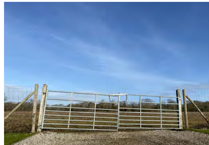
7. East Entrance of Site from access to crematorium
