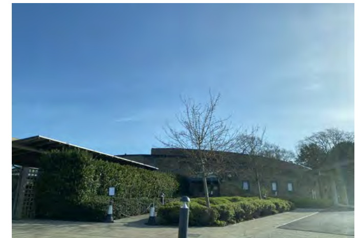
9. View of Crematorium located North West of Site
