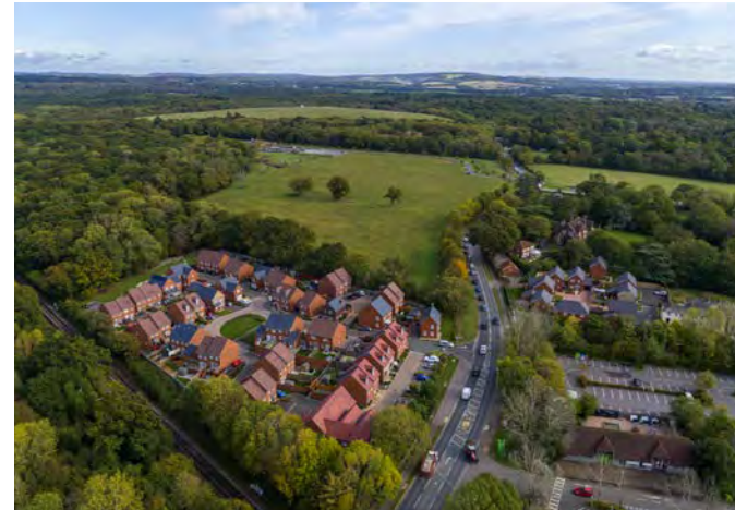
1. South West view of Site from Bartons Road
