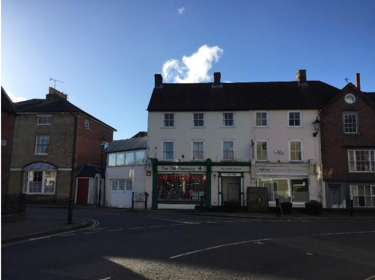
Figure 9: Important visual stop at the west end of Queen Street.
