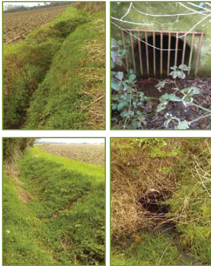
Figure 3.9: Photographs of Land Drainage Network
