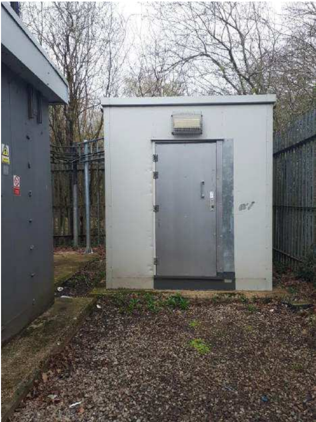
Plate 16: Building units associated with telecommunications mast.
