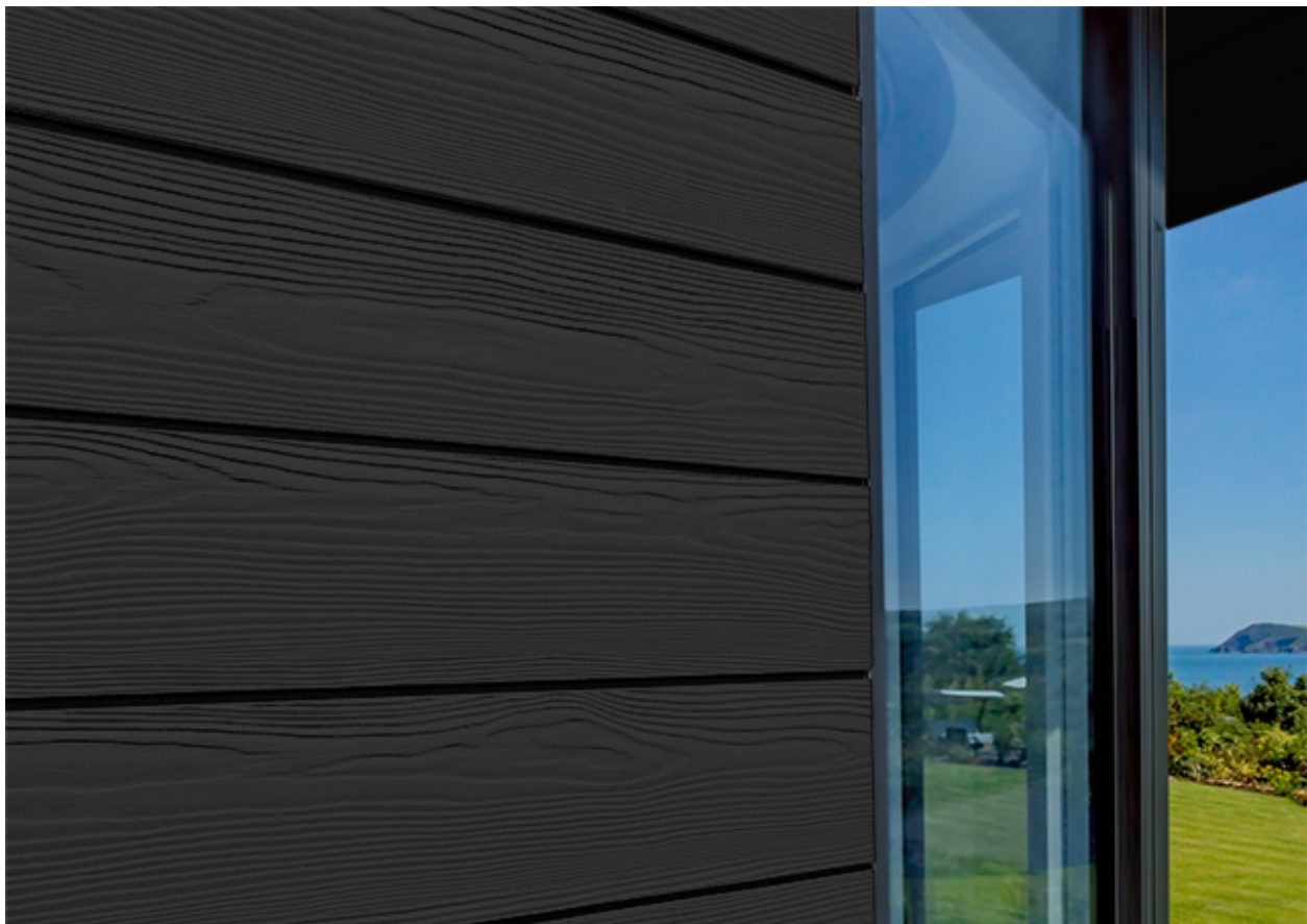
Walls: Timber Cladding
