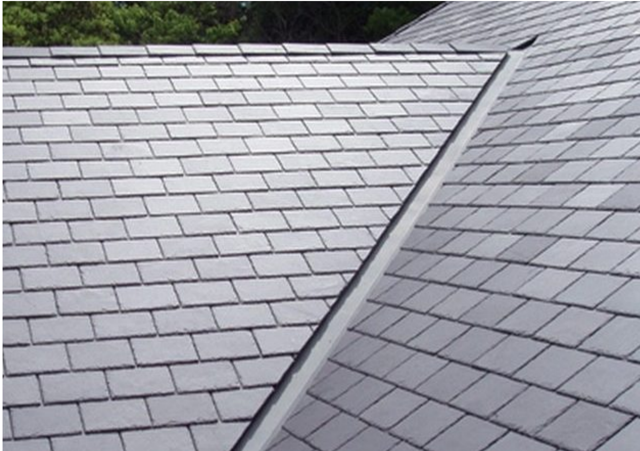
Roof: Slate Tiles
