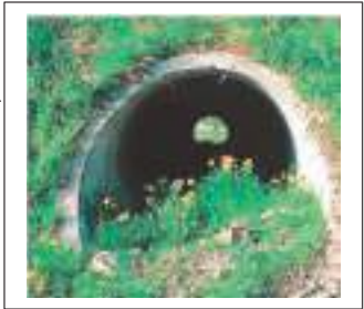
If pathway along eastern boundary created, a small ‘wildlife’ culvert will be required to go underneath it to maintain habitat connectivity.
