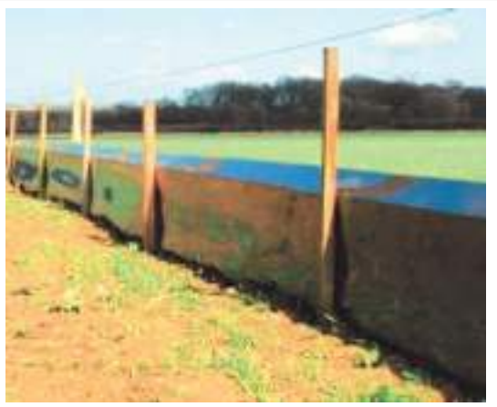
1 mm HDPE semi-permanent reptile fence used along edge of the retained receptor. This will need to be installed around the entirety of the site although it’s exact location will need to be agreed with land surveyor to ensure there is adequate working space during construction.
