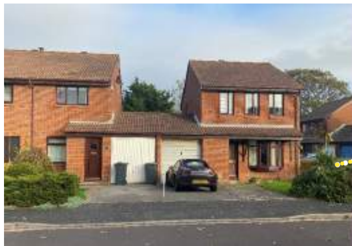
Exiting Buildings within the site
