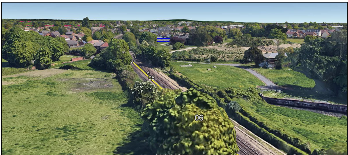
Figure 14 View towards proposed development from train driver receptors 4-6 – 3D aerial image
