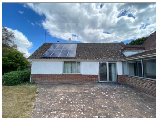
Figure 8 – Western elevation of the rear extension
