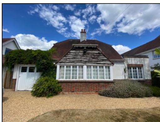
Figure 6 – southern elevation of the house and adjoining garage
