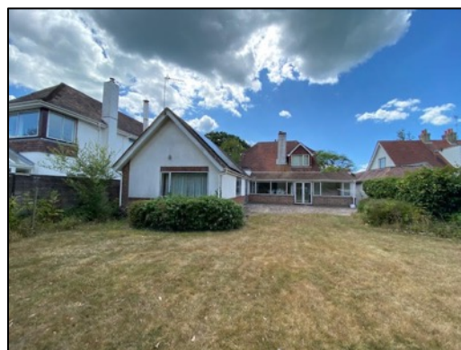
Figure 7 – northern elevations of the house
