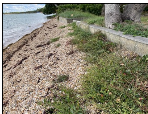
Figure 5 – sea wall at the northern boundary of the property
