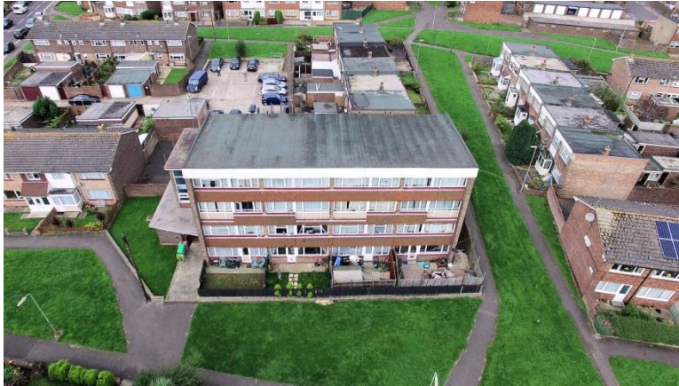
Photo 1 - Arial view of the block (Front Elevation)
