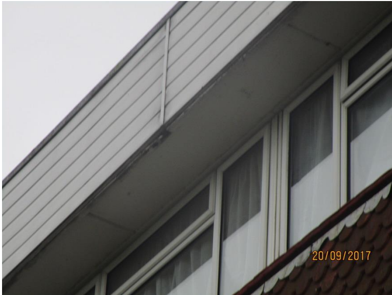
Photo 4 - Existing Facia Board and Soffit
