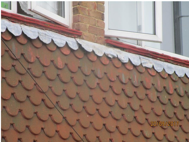
Photo 5 - Tile hanging to front elevation
