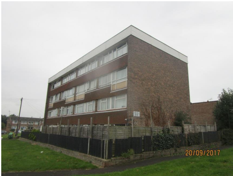
Photo 2 - Front Elevation showing boundary fencing
