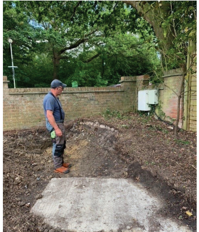
Image showing difference in ground level (approximately 1 metre) between the site and Highway land at boundary adjacent to oak. The existing concrete slab foundation is also visible at the reduced level of the proposed garage building
