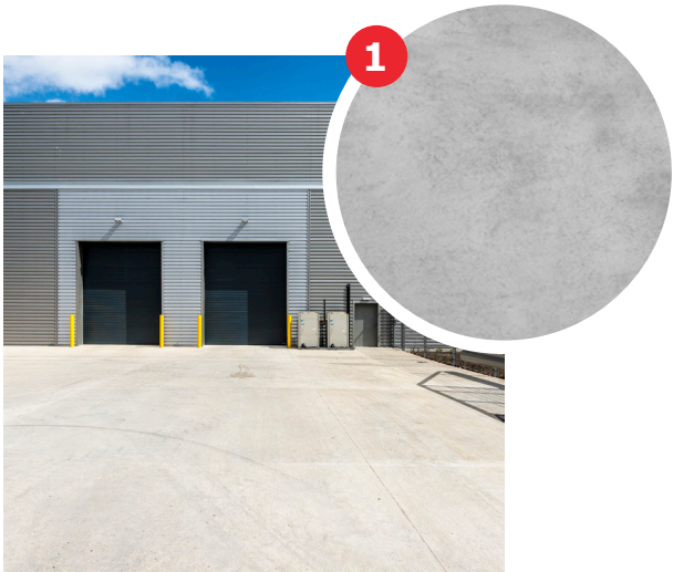
Yard: in Concrete (1)
