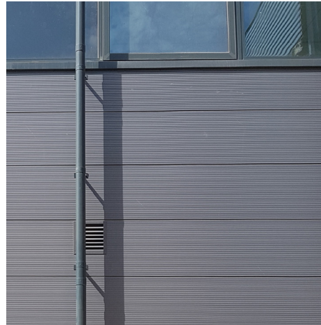
Horizontal Cladding: Composite Panels in Anthracite RAL 7016 (1)
