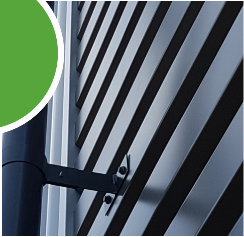
Rainwater Pipe: PPC Aluminium in Merlin Grey RAL 180 40 05 (2)
