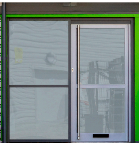
Entrance Doors & Windows: Aluminum Framed System in Merlin Grey RAL 180 40 05 (2) with Metallic Silver RAL 9006 (3) Door Frame
