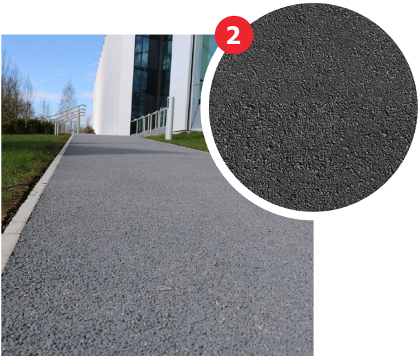
Access Road: in Tarmac (2)
