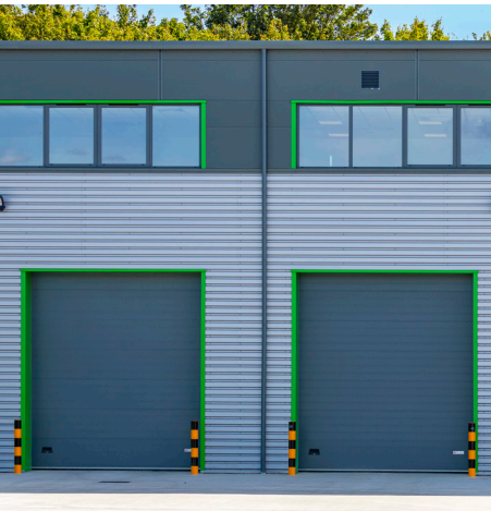
Loading Doors: Industrial Sectional Doors in Merlin Grey (2)
