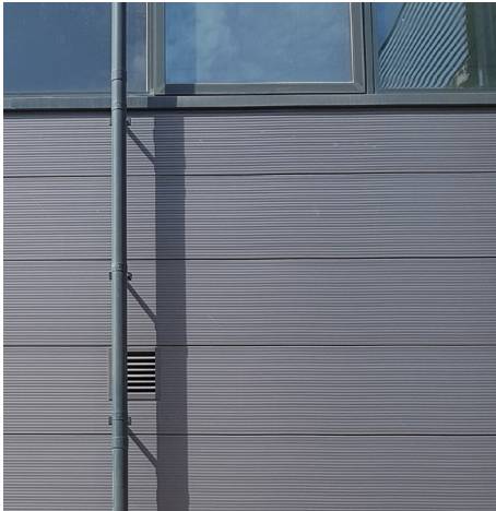
Cladding: Horizontally laid, micro-rib, composite cladding in HPS200 Ultra Merlin Grey (2)
