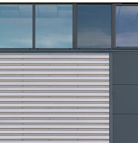
Entrance Doors & Windows: Aluminum Framed System in Merlin Grey RAL 180 40 05 (2) with Metallic Silver RAL 9006 (3) Door Frame
