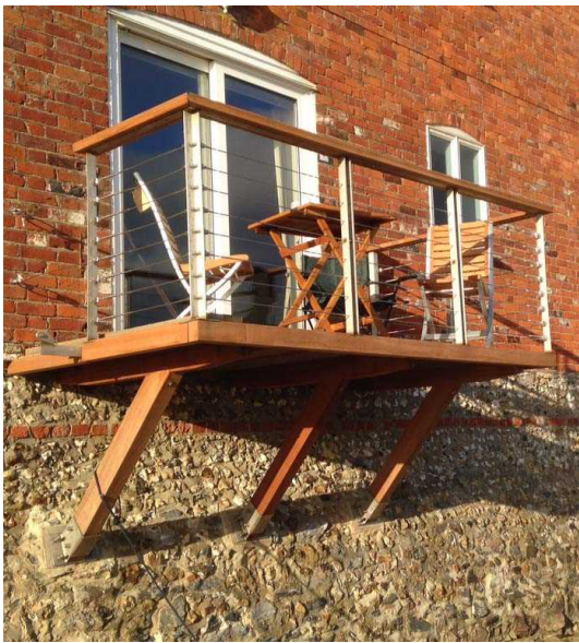
EXISTING BALCONY SHOWING STAINLESS STEEL AND HARDWOOD USED IN COMBINATION. SIMILAR PRINCIPLES OF CONSTRUCTION ARE PROPOSED FOR THE BRISE SOLEIL
