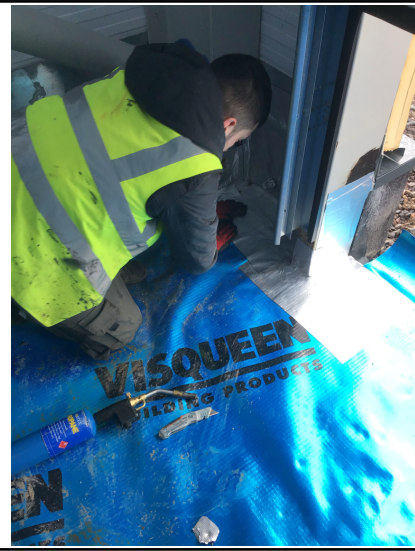
Installers have patched
