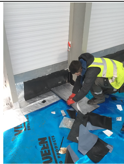
Installers sealing steel columns.
