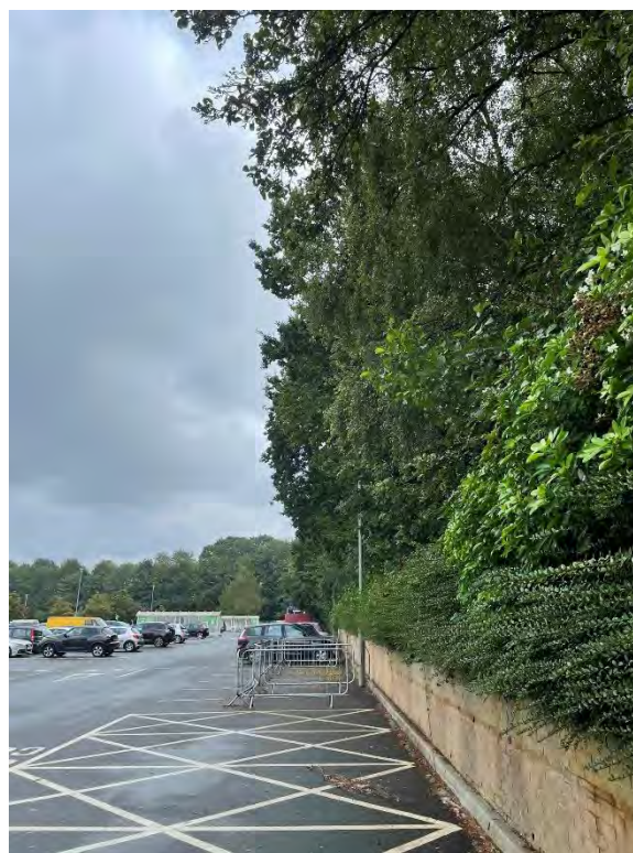
Photo 2 – Another view of G1, mixed deciduous woodland above the 1.2m high brick retaining wall showing the canopy overhang
