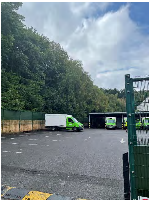
Photo 3 – View of G2, mixed deciduous woodland above the 1.8m high brick retaining wall with welded mesh fencing around delivery van parking and loading area
