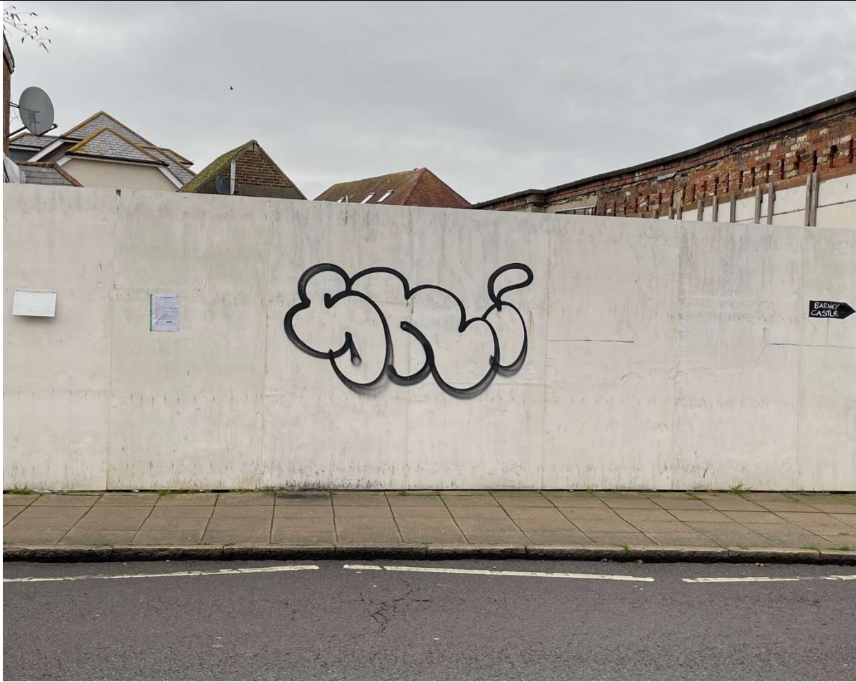
Figure 4: Front elevation of 5 & 7 East Street.
