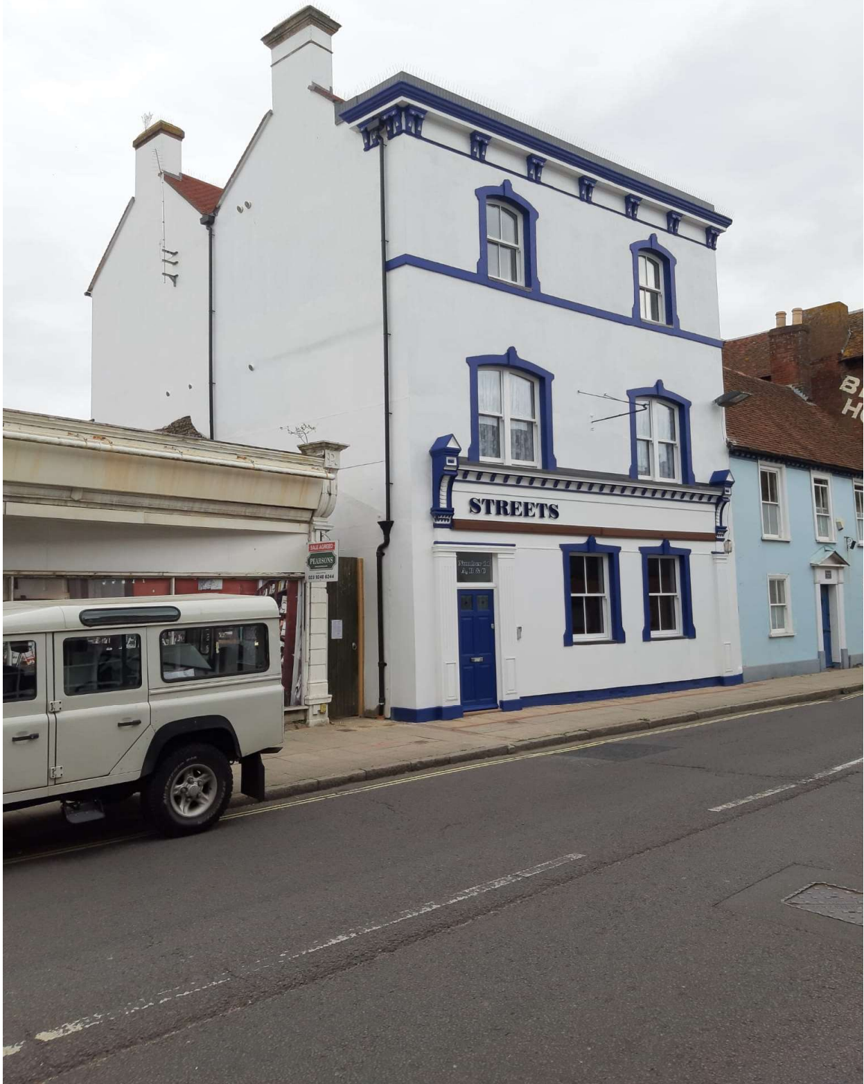
Figure 2: Front elevation of 9&11 East Street.
