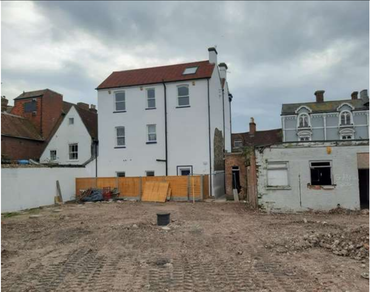
Figure 3: Rear elevation of 9 & 11 East Street.
