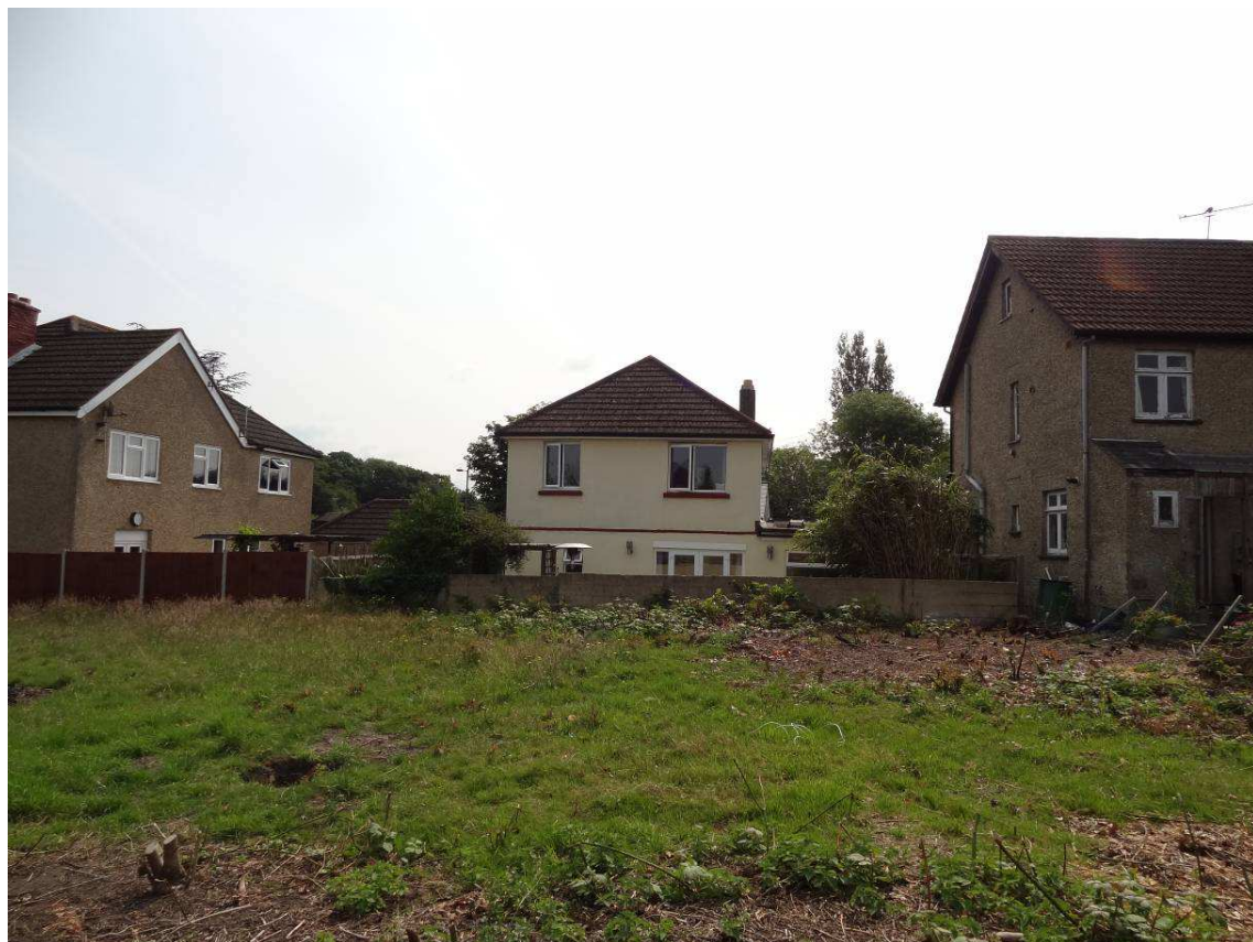
Photo 14 – View towards rear of No.165 Park Avenue on eastern boundary of site.
