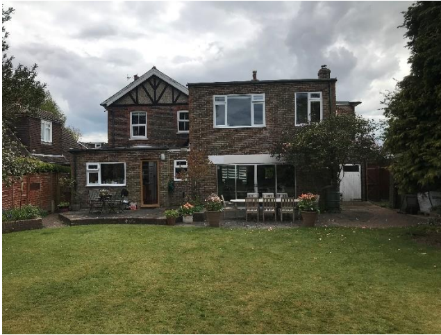
Figure 3: Rear Elevation of dwelling
