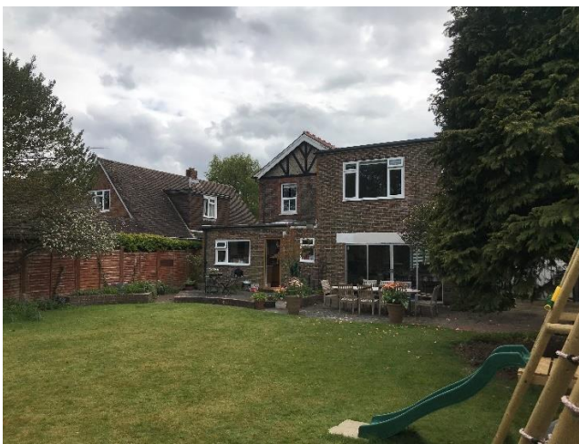
Figure 4: Rear of 28 Park Crescent, with no. 28a in view to the East
