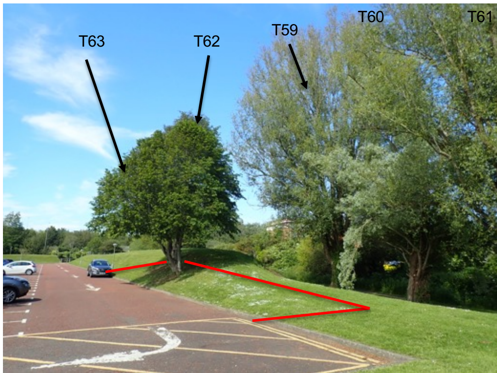
View to north along existing berm. The berm is to be excavated back and re-profiled to allow extension of the car park. Lime trees T62 and T63 to be removed. Within the root protection area of T59, T60 and T61, in the area indicated in red, there must be hand dig excavation and the cut back area of the berm must be retained by a supporting structure, rather than re-profiled.
