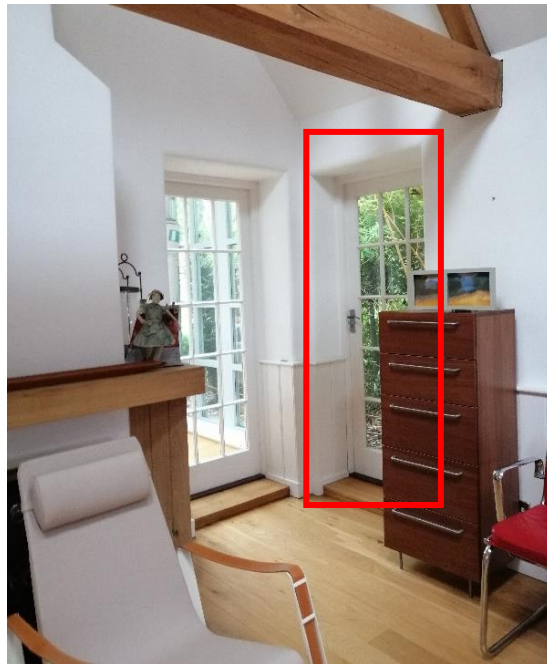
Figure 6, Existing timber door to be replaced with a single aluminium framed window
