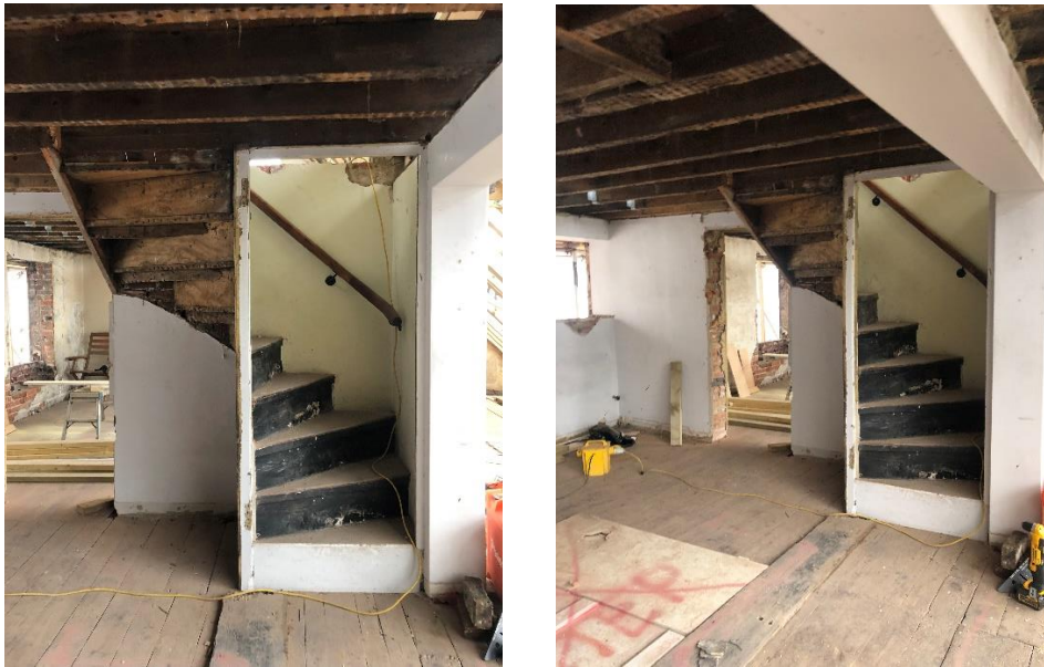
Figures 7&8: Staircase to first floor Hall.
