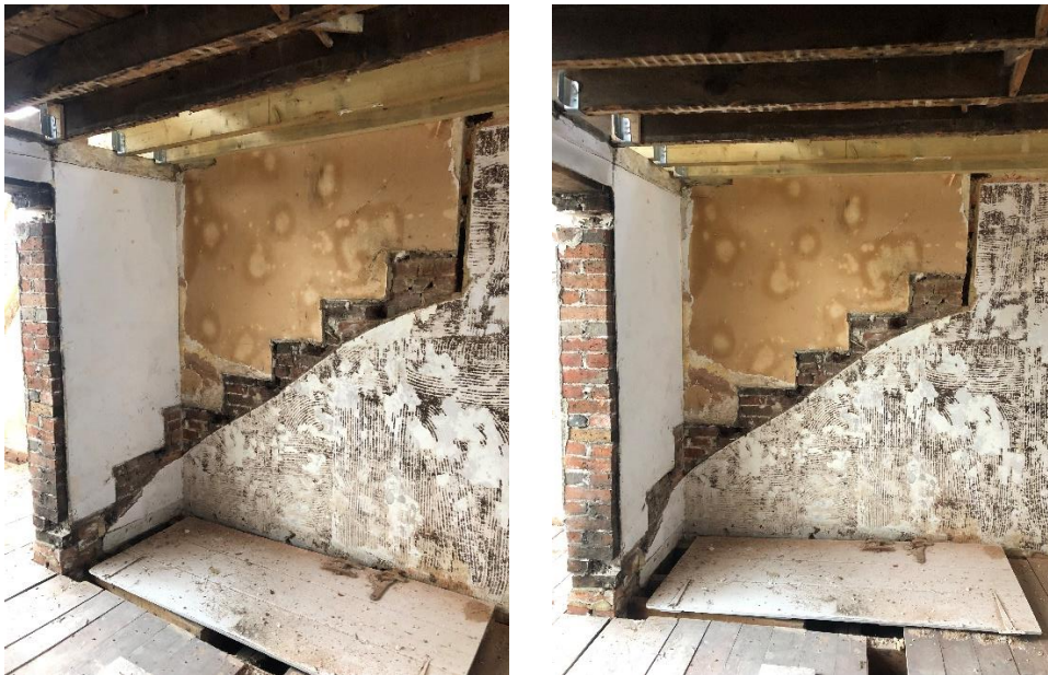
Figures 5&6: Staircase in Bedroom 1 removed.
