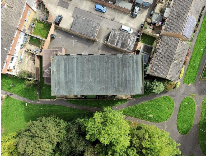
Photo 1 - Arial view of the block
