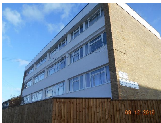
Similar Completed Pilot Block (Prospect Lane)
