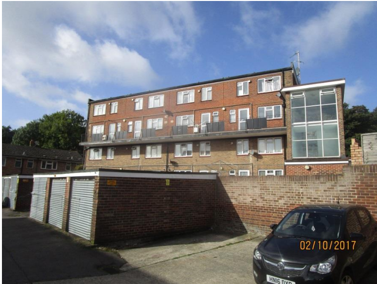
Photo 3 - Rear elevation showing balcony walkway
