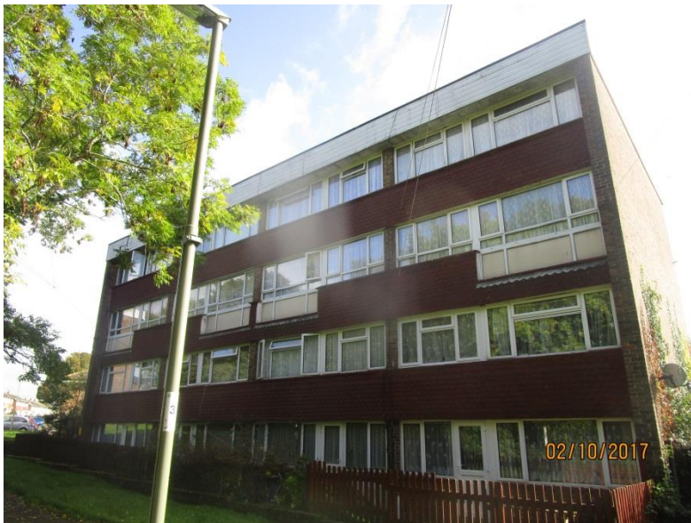
Photo 2 - Front Elevation showing boundary fencing
