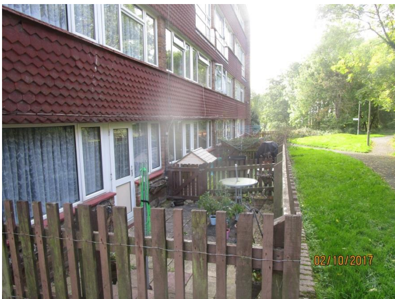
Photo 5 - Tile hanging to front elevation
