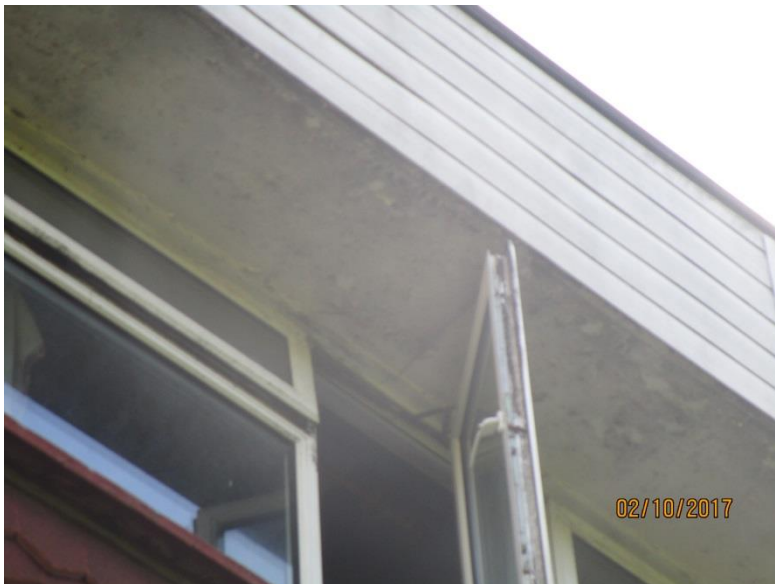
Photo 4 - Existing Fascia Board and Soffit
