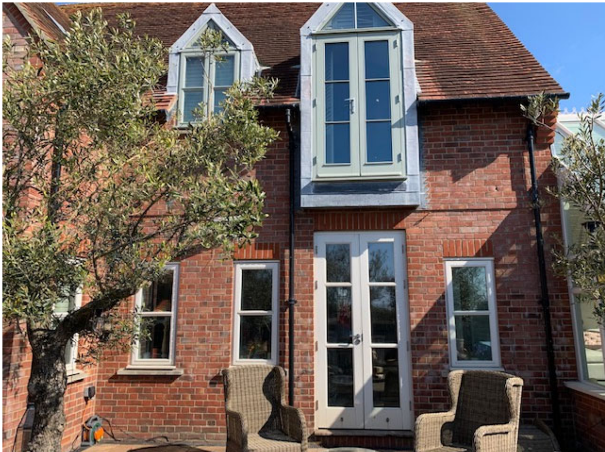
Plate I : Tower House– South Elevation showing area of proposed balcony
