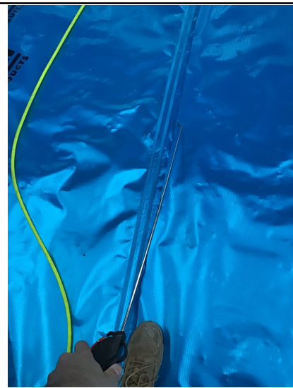
Air lance test being carried out.
