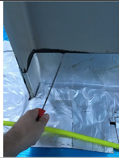
Pick and probe test to steel column
