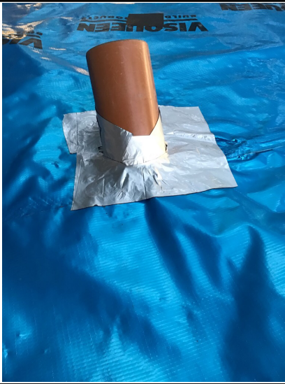
Large pipe penetration sealed to
