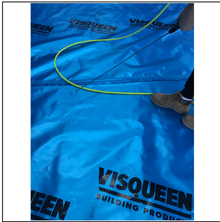
Air lance test again being carried out.
