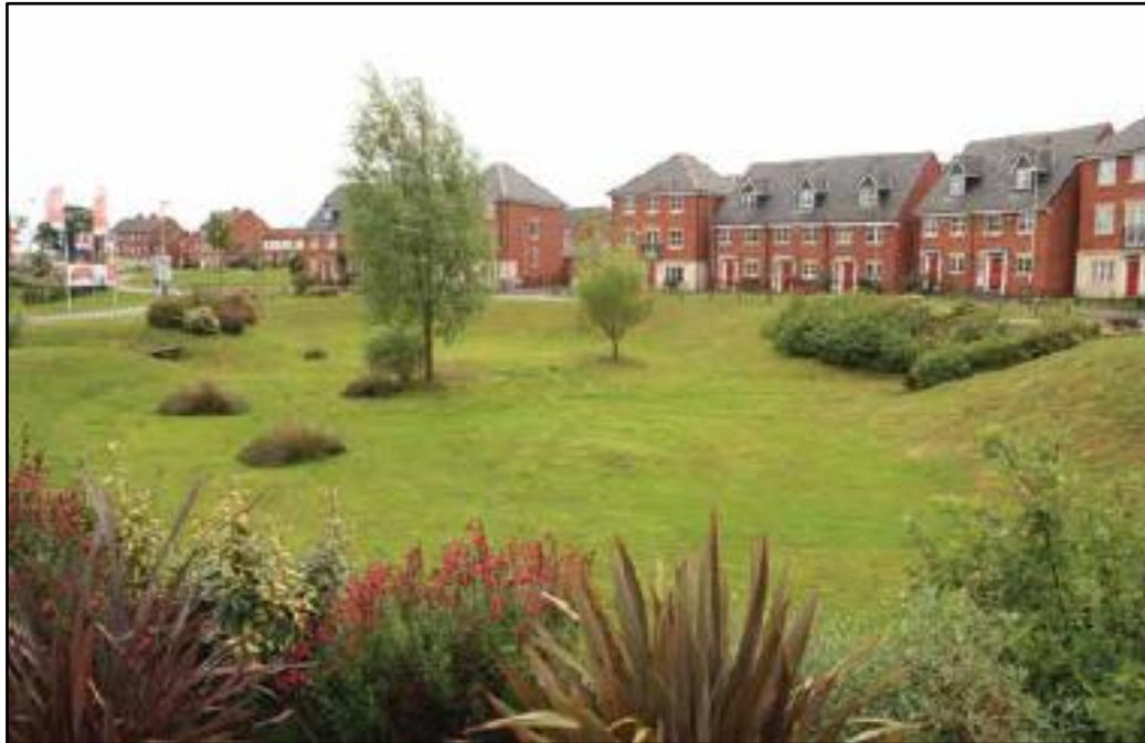
Figure 5: Example of a detention basin serving a housing development (Source: Ciria C753)
