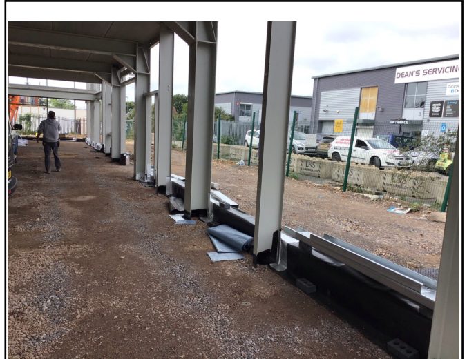
Overview photo shown the completed
