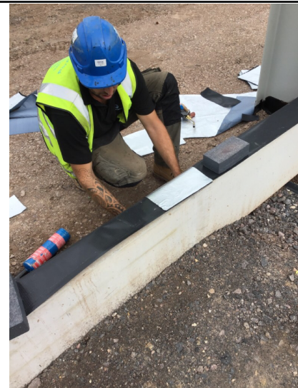
Installer carrying out work to dpc
