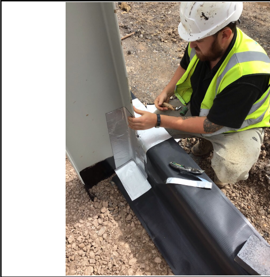
Installer carrying out works to perimeter
