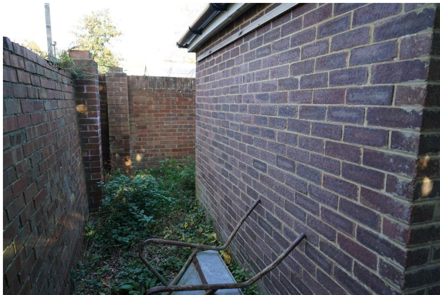
Fig.4: View looking at the rear west end of the garage and perimeter walls
