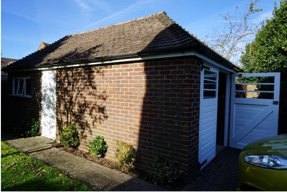
Fig.5: View looking at the south elevation of the garage.
