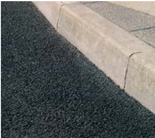
ASPHALT SURFACE TO MAIN ACCESS ROAD
