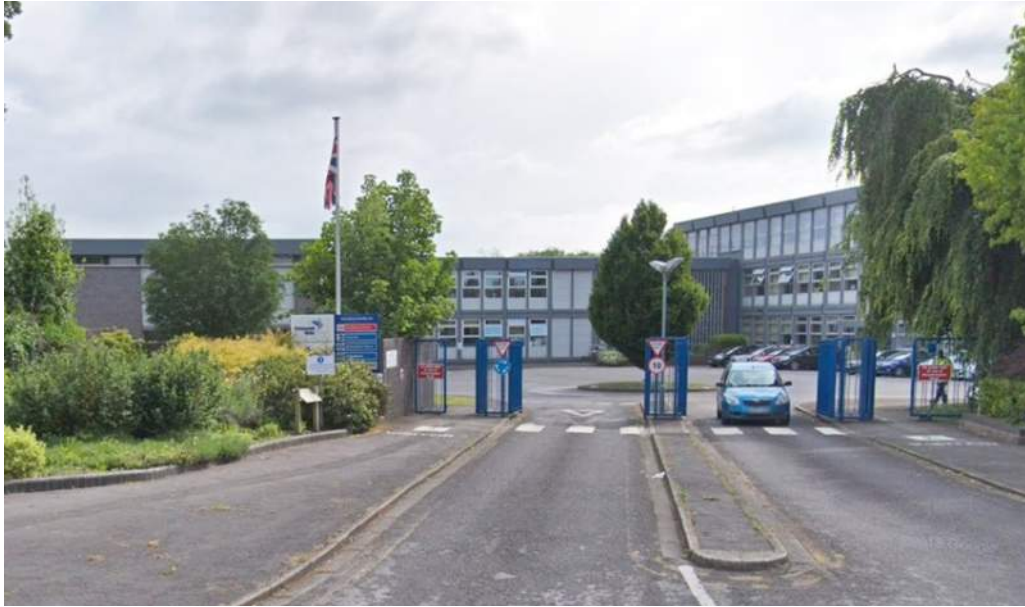
View of existing Portsmouth Water building from front entrance
