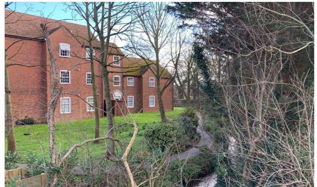
Manor Court Flats off Brockhampton Road
