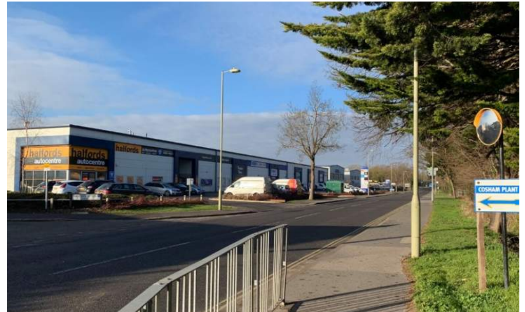
Trade counter units—view from Solent Road/ Brockhampton Lane
