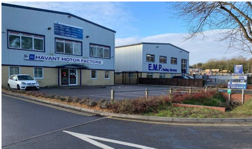
Industrial estate—view from Solent Road opposite site entrance
