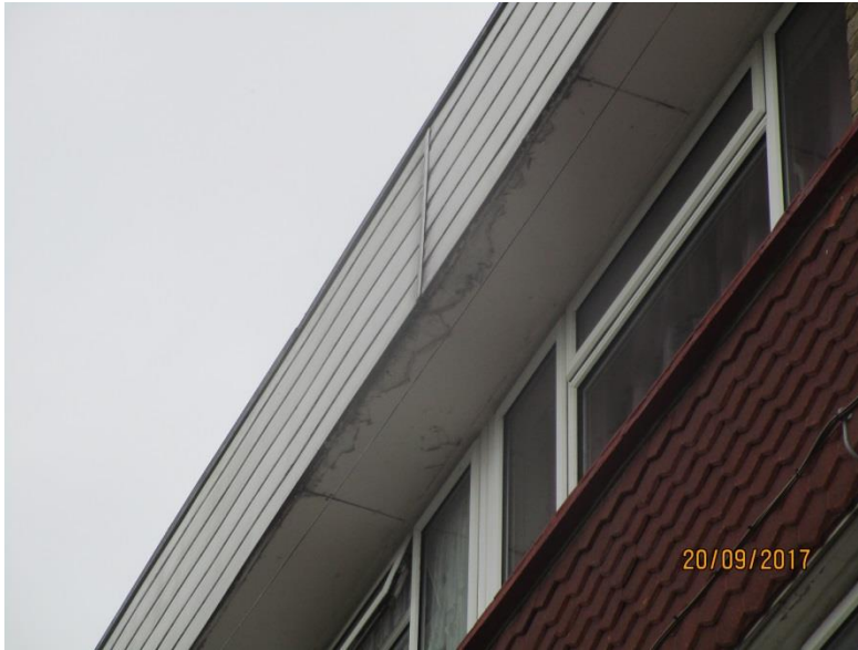
Photo 4 - Existing Facia Board and Soffit
