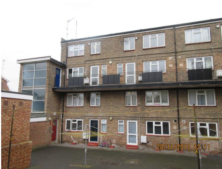
Photo 3 - Rear elevation showing balcony walkway
