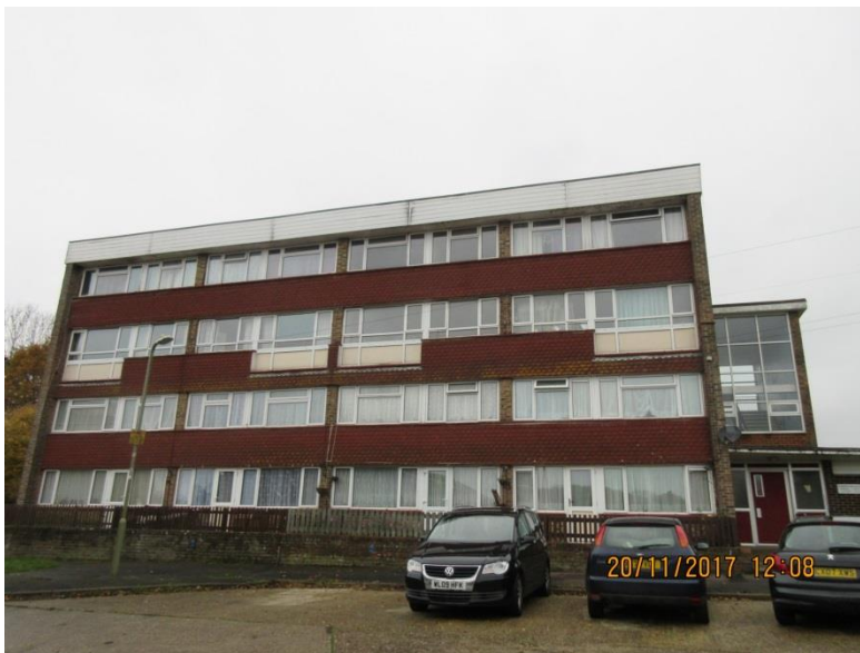
Photo 2 - Front Elevation showing boundary fencing
