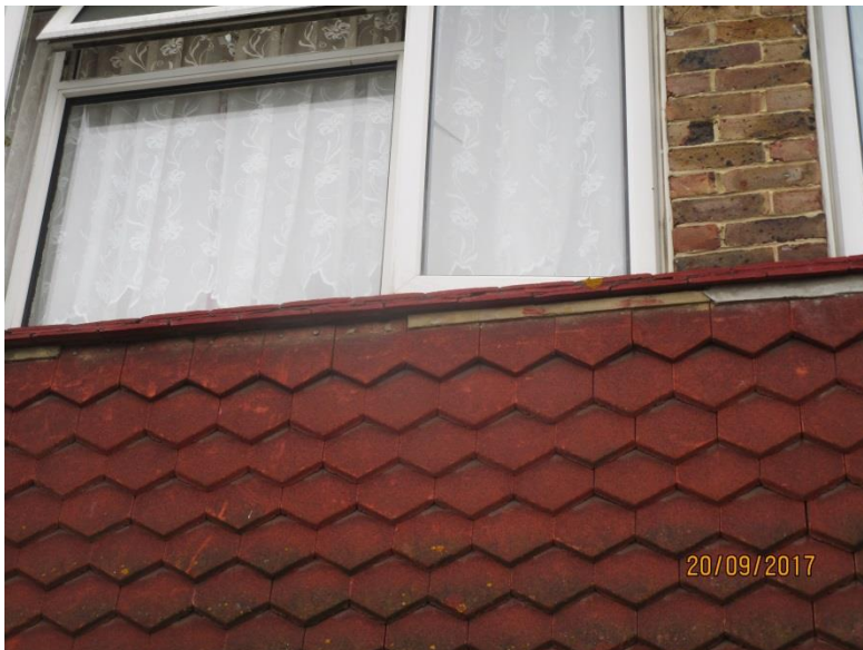
Photo 5 - Tile hanging to front elevation
