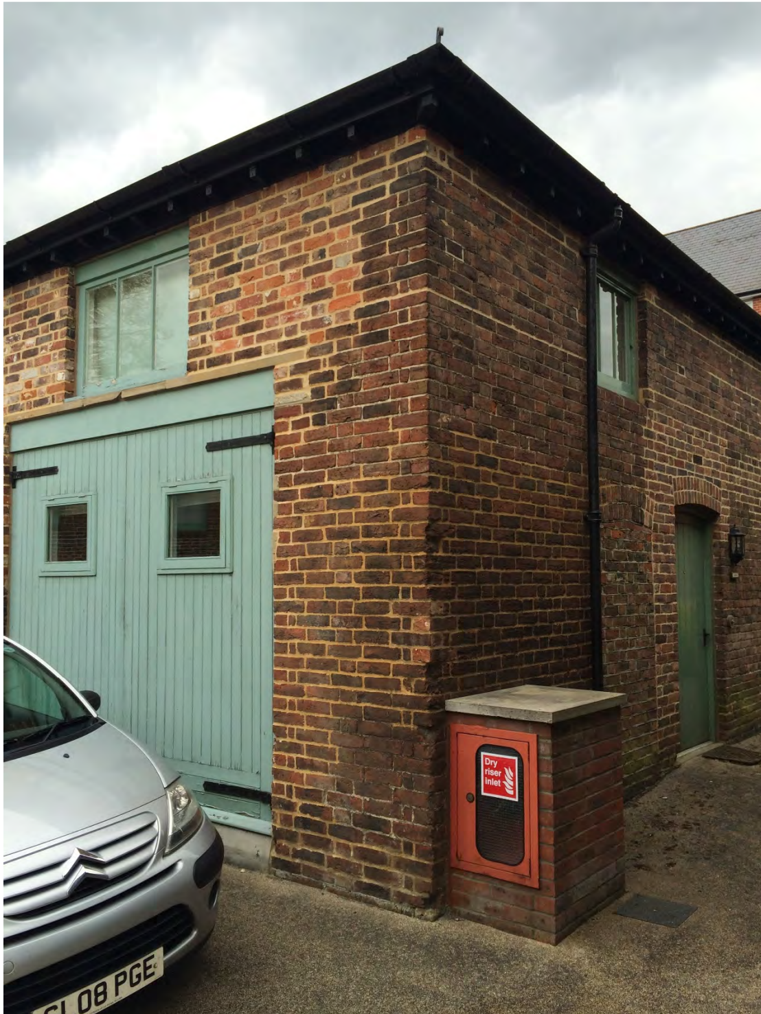
Guest Suite – Part of original construction and not to be effected by the window replacement works.
