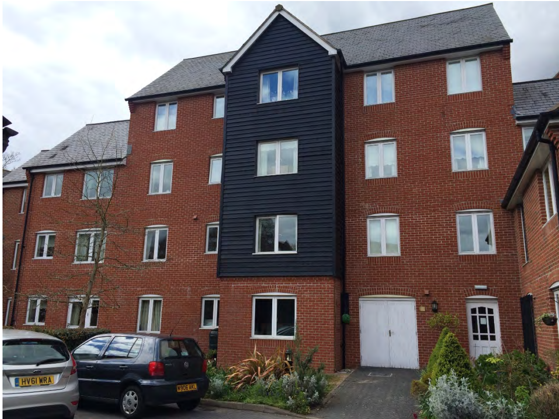
East elevation viewed from car park
