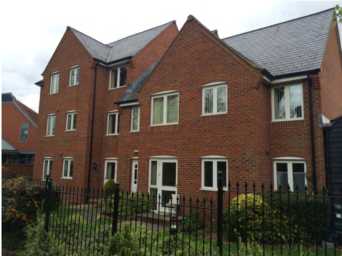
South Elevation – Including both doors and windows to be replaced.
