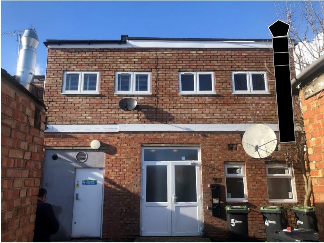
Rear view of the building with equipment showing in black
